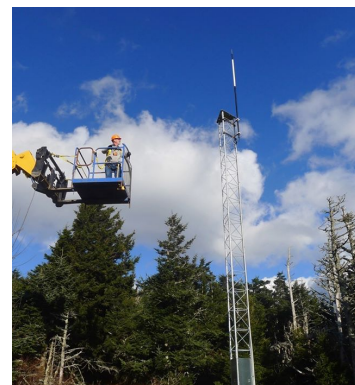
MM Radio Tower: John Whitehouse rides a lift to install and adjust the antennae on a Traveler Information Radio Station tower that High Peaks helped Mt. Mitchell State Park purchase and install in 2019
