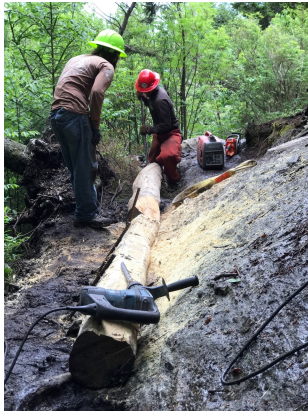
AmeriCorps workers from the American Conservation Experience trail-building crew installing a crib on the Mt. Mitchell Trail in 2017, work funded by grants obtained by High Peaks
