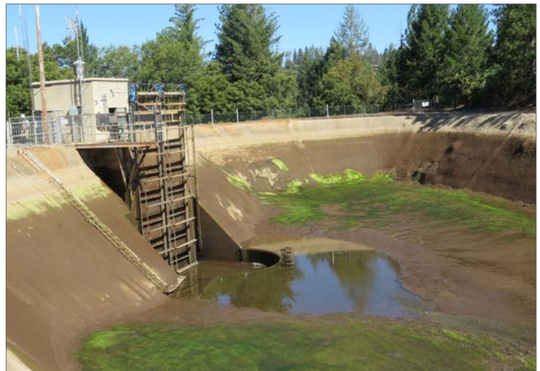
Photo: Existing site conditions.
