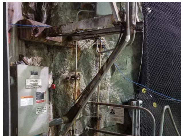
Photo: Existing site conditions.
