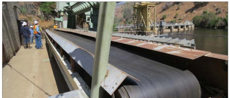
Photo: Existing site conditions.
