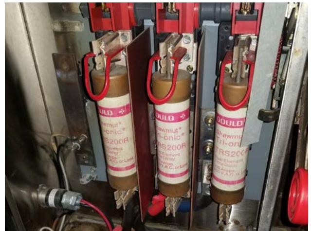
Photo: Existing site conditions.
