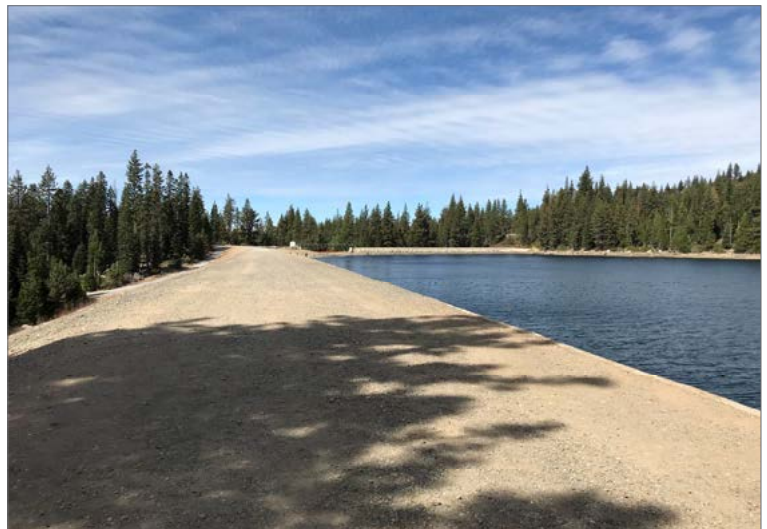
Photo: Existing site conditions.
