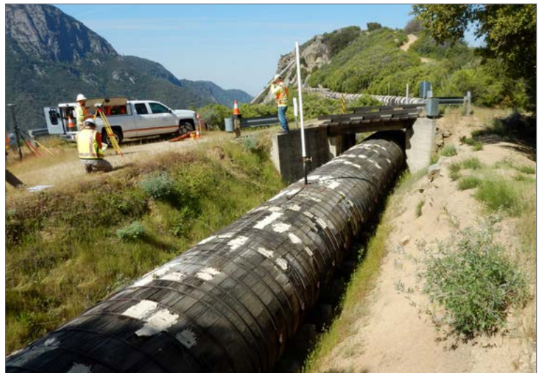
Photo: Existing site conditions.
