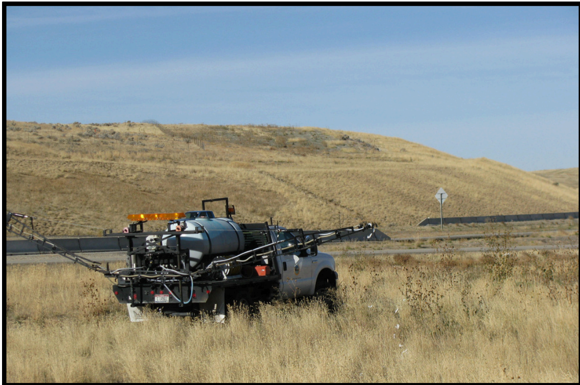
Photo: Idaho DOT
