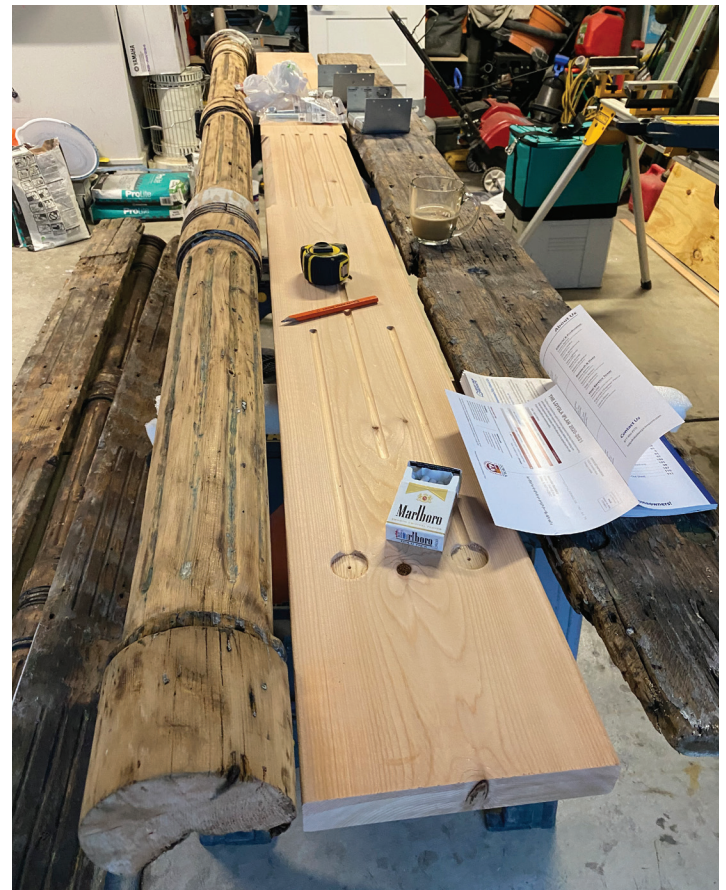
Façade columns of 1720 N Sedgwick being replicated (photo by Burt Richmond, 2020)
