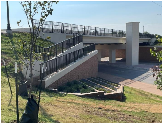
Bridge railings are complete
