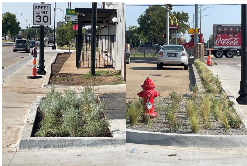
Planting of landscaped beds continues
