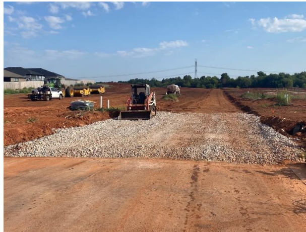
Flint Hills Addition Section 2 – Rough Grading
