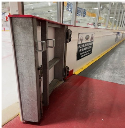
Bleacher Face Board in the alleyway in front of the bleachers
