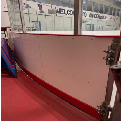
Front Face Boards near the rink access door
