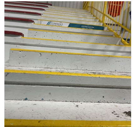
Stair riser on bleachers
