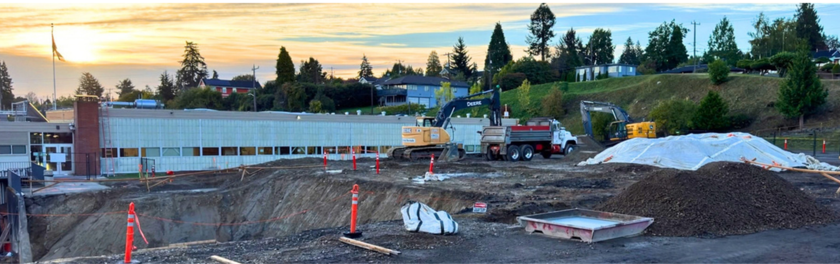
Foundation work is underway as the Norcliffe Academic Center, Cristo Rey Jesuit Seattle's permanent academic home, takes shape.
