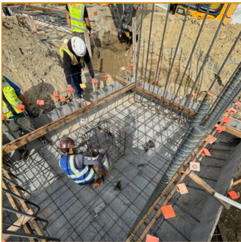
Steel reinforcement and foundation work
