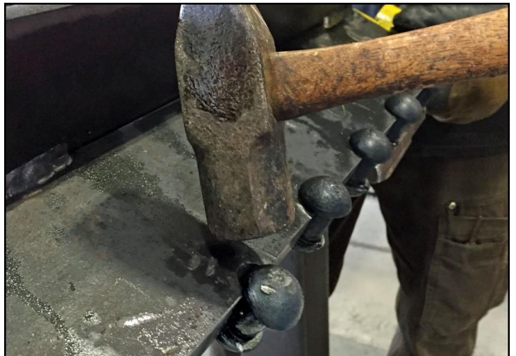
Rivets are removed with a few blows with a hammer
