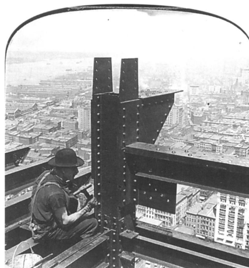
Figure 20. A rivet tester followed along after the riveting crews and used a special hammer to check for loose or dull-sounding rivets. Photo courtesy R. M. Vogel.
