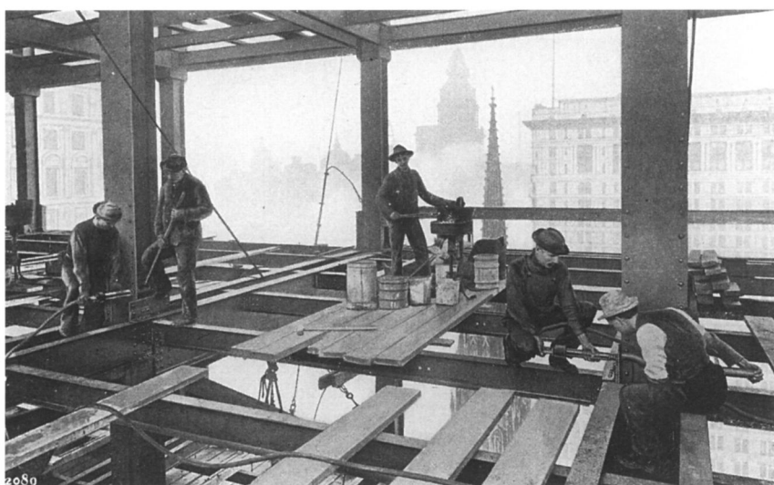
Figure 23. A turn-of-the-century Ingersoll-Rand Company catalog showed pneumatic hammers in use on the construction of the Trinity Building in New York. It also illustrated a variety of holders-on, some more or less devised on the job. The second man from the left uses a heavy sledge and his foot wedged between the flanges of the column as a holder-on, while the man on the right holds a piece of pipe whose end has been bent to allow alignment with the end of the rivet. The forge boy or heater, surrounded by barrels of rivets, stands ready to toss the next hot rivet to one of the riveting gangs.
