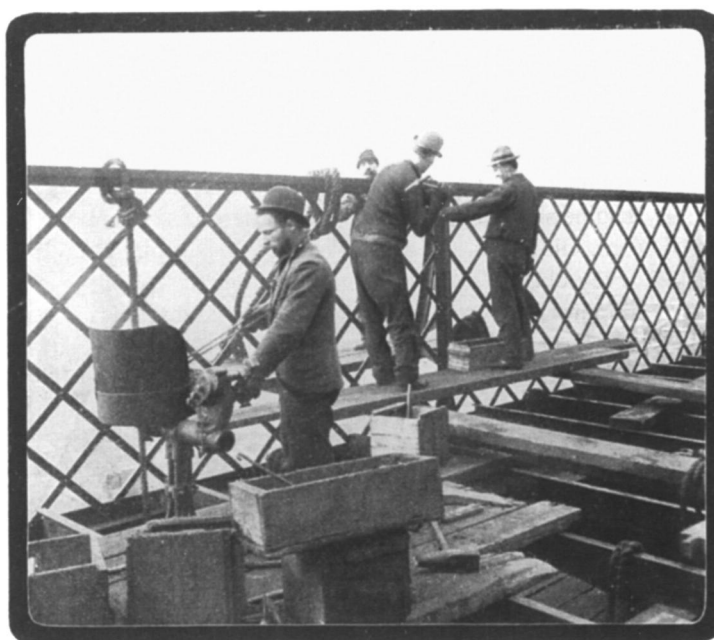
Figure 2. This four-man crew is field riveting a bridge railing. The man in the foreground operates a forge with a hand-cranked blower to heat the rivets. He tosses the rivets to the man on the far right, who catches them in a special bucket and then places them in the rivet hole. The man on the far side of the railing holds a dolly bar on the already formed head of the rivet, while the man with the hammer shapes the other end of the rivet into a head. The size of the hammer suggests that, as would be expected, the rivets on the railing were relatively small. Frank Leslie's Popular Monthly 52 (July 1901): 272.
