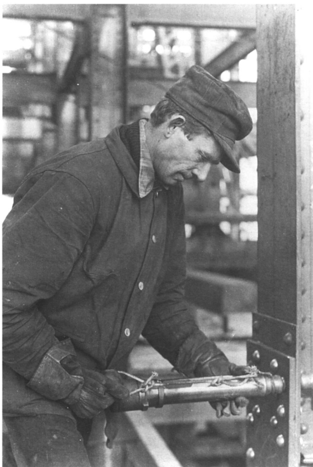
Figure 18. Lewis W. Hine photographed a riveter working on the Empire State Building in 1931. The force of repeated blows on the riveting cup tool necessitated ad hoc ways of keeping it on the end of the hammer. This man used a simple rope. Photo courtesy of the George Eastman House.
