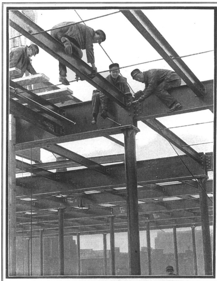
Figure 1. A 1901 article on structural workers included this illustration of iron workers bolting up a skyscraper framework. Frank Leslie's Popular Monthly 52 (July 1901): 263.
