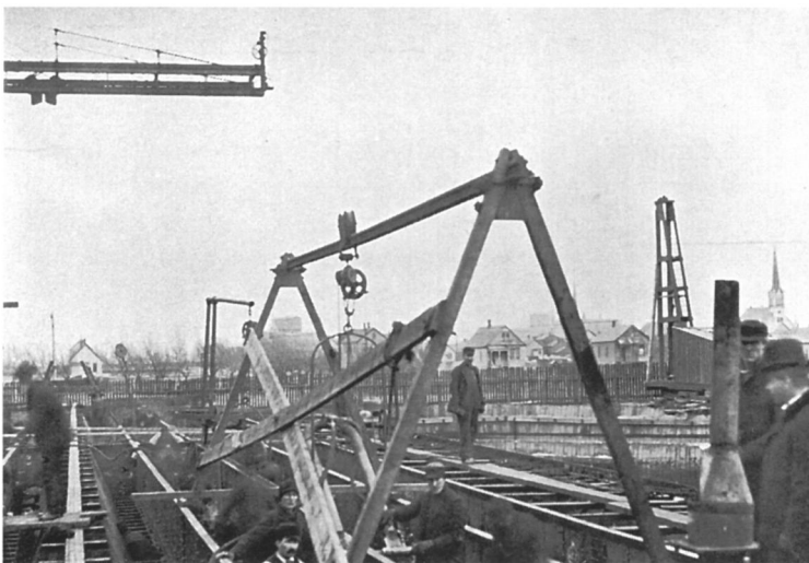
Figure 16. Ultimately the work required yoke riveters large enough to necessitate, even in the context of a shipyard, a special A-frame and rigging to handle and operate them. The yoke riveter is parallel to the X-bracing of the A-frames. The lighter bow frame above it is part of the rigging hanging from the rail between the A-frames. W. I. Babcock, "Portable Pneumatic Riveters in Shipbuilding," Transactions, Society of Naval Architects and Marine Engineers 6 (1898), plate 46.
