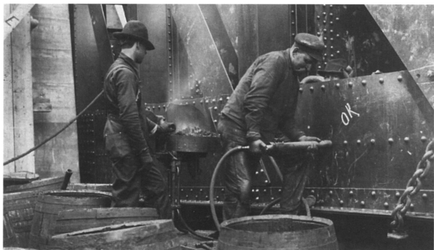
Figure 22. If the construction of the Peterborough Lift Lock in 1902 on the Trent-Severn Waterway in Ontario is any indication, pneumatic riveting hammers were much more readily adopted in Canada than in Europe. Photo courtesy of Parks Canada.
