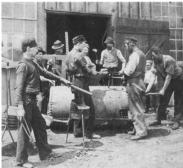
Figure 5. Boilermaking in general but riveting in particular required a highly skilled workforce and was physically demanding. This shop operation used a large hand-powered bellows connected to a very small forge for heating the rivets. The man on the far right holds a bar inside the boiler to back up a rivet, while the two men in foreground with hammers are in position to form the head. Those in the background hold a variety of squares, hammers, and tongs used by riveters. Photo courtesy R. M. Vogel.
