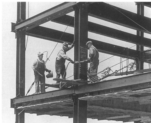
Figure 19. Hine's photographs of the Empire State Building construction included this view of a three-man riveting crew. The man on the left caught the red-hot rivet in his special bucket and placed it in the hole with his tongs; the next man held it in place, in this case with a pneumatic holder-on; and the third man operated the riveting hammer. Photo courtesy of the George Eastman House.
