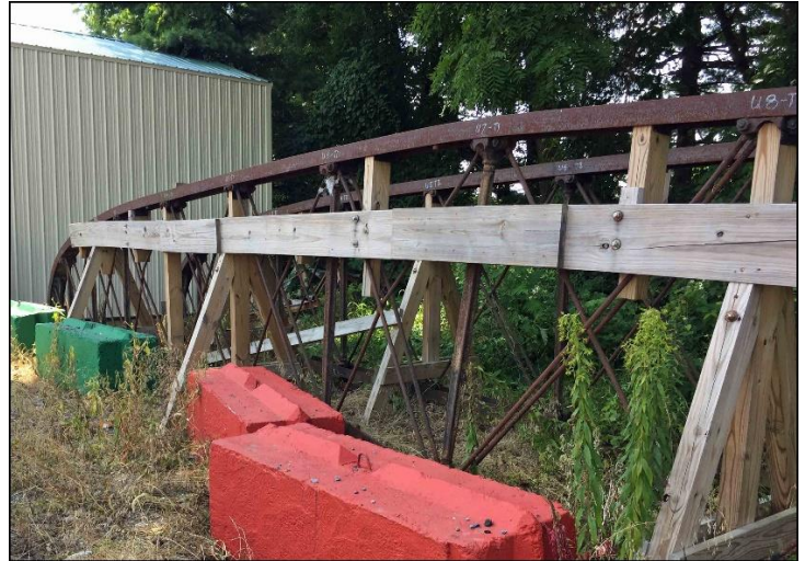
Tank Farm Road Bridge at the City of Bethlehem Public Works storage yard
