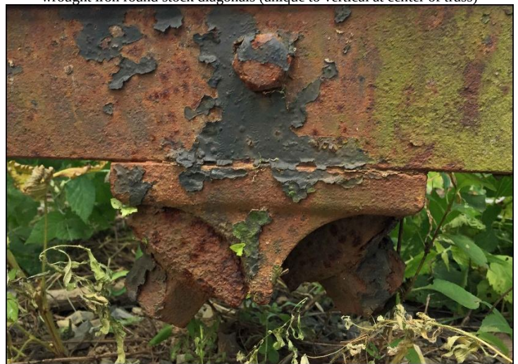
Lower chord cast iron bolted diagonal connection
