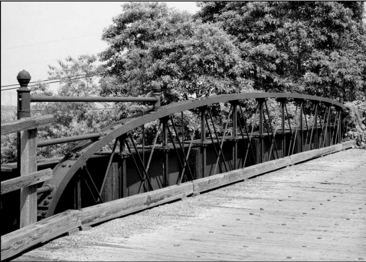
Tank Farm Road Bridge crossing Reading Railroad tracks Emmaus, Lehigh County, PA. Photo: HAER PA123
