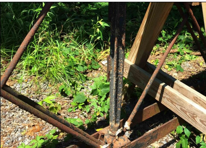
Lower chord cast iron connection with a friction fit cruciform vertical post and wrought iron round stock diagonals
