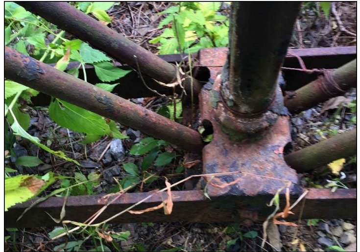
Lower chord cast iron connection with a friction fit cruciform vertical post and wrought iron round stock diagonals (unique to vertical at center of truss)
