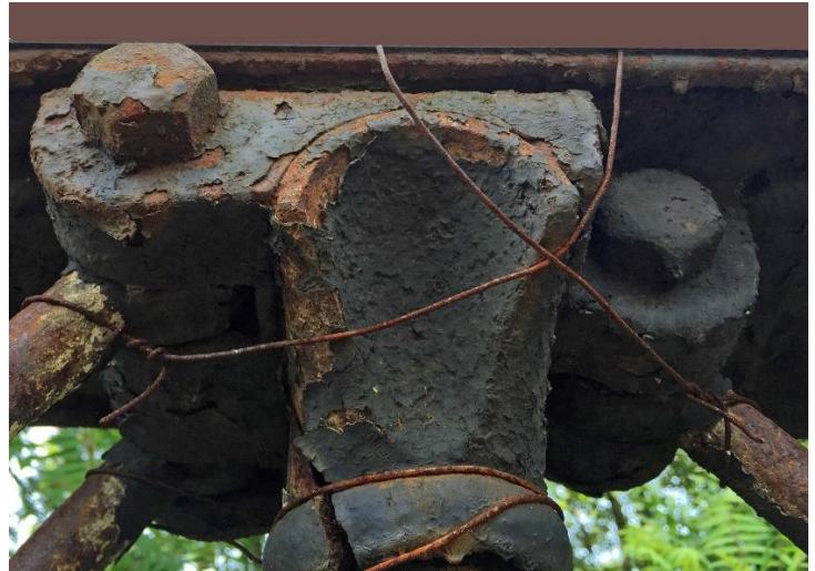
Upper chord cast iron rocker assembly
