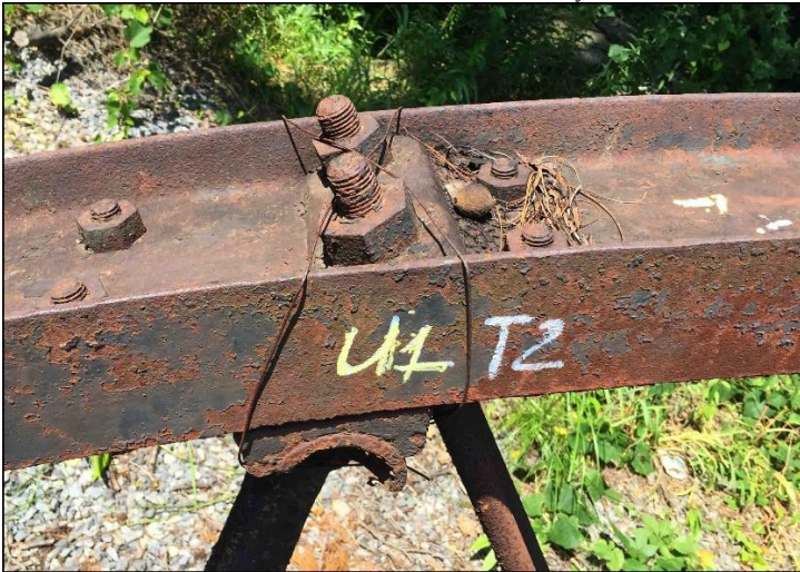
Upper chord bolted cast iron connection
