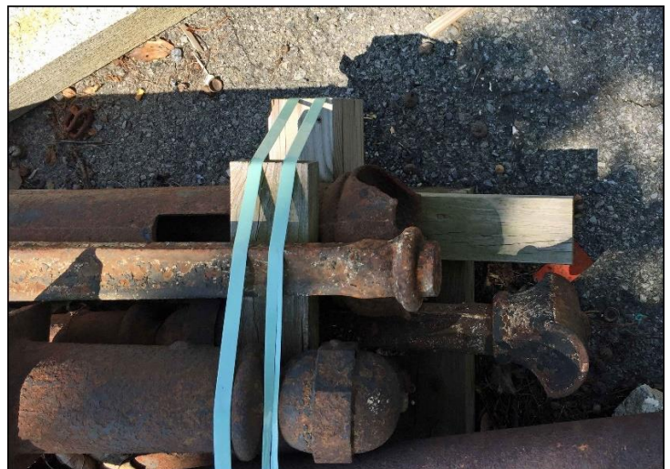
Palletized cast iron sections. Center of photo: friction fit cruciform vertical post end
