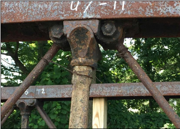
Upper chord cast iron bolted connection with a friction fit cruciform vertical post attached to a cast iron rocker assembly
