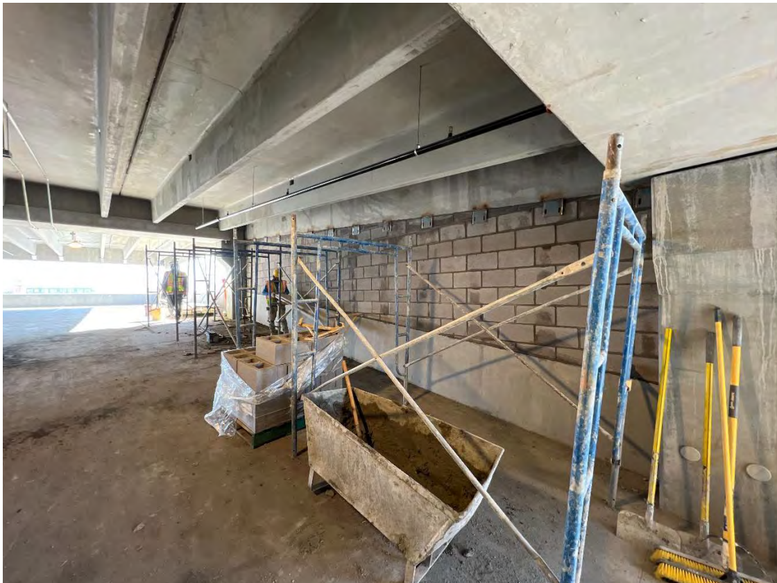
Garage CMU Infill Completed
