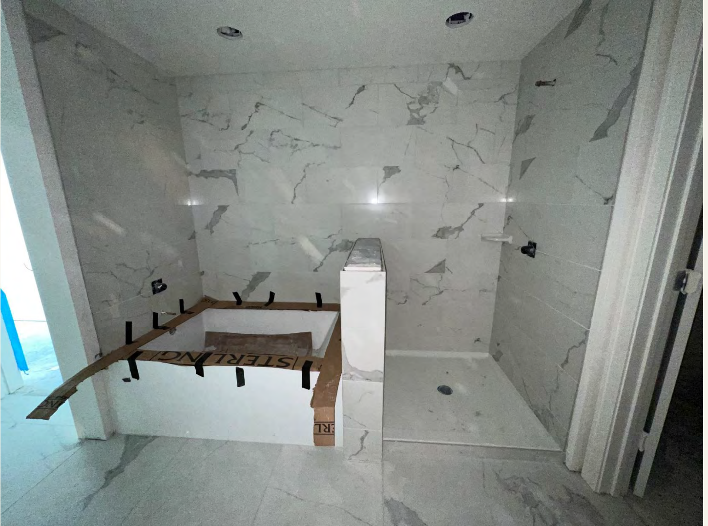
Description: Level 9 – Mockup Tile Surrounds Complete.
