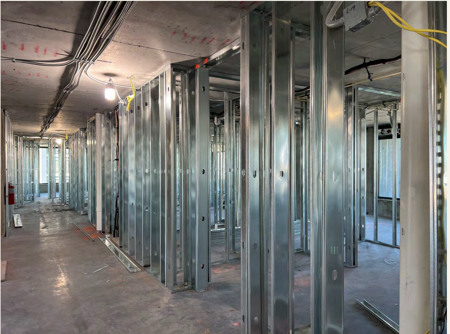
Description: Unit Wall Framing in progress on Level 19.
