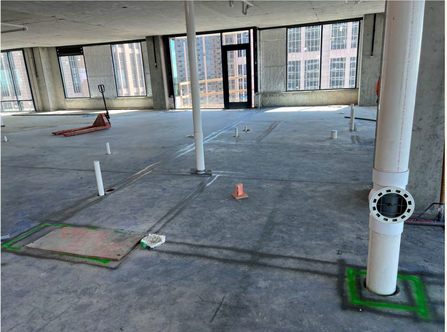
Description: Unit Wall layout in Progress on Level 21.
