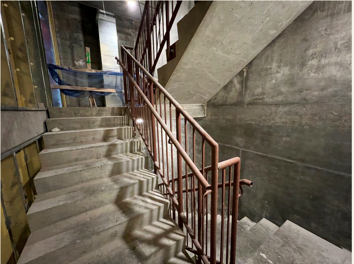
Description: Metal Stair Railing Installation in Progress.
