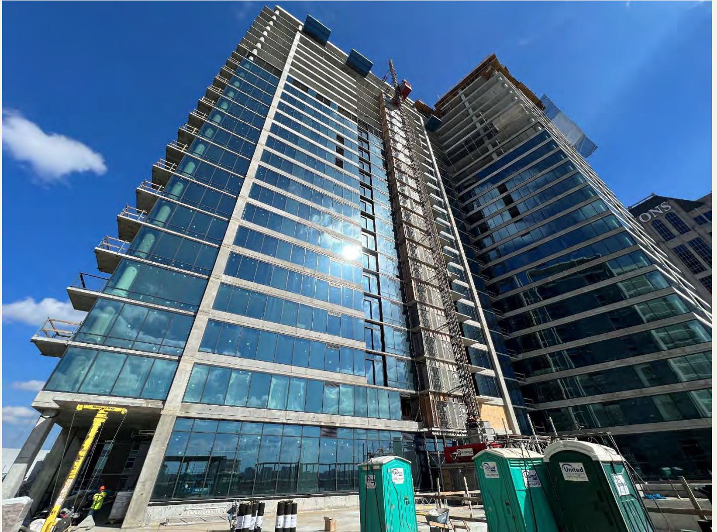
Description: West Elevation of Site – Exterior Glazing in Progress.
