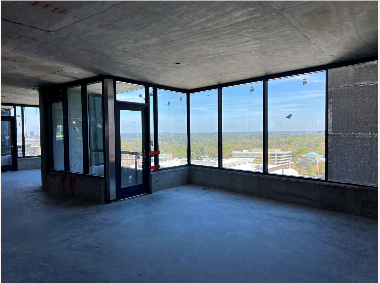
Description: Window Wall Glazing Installation Complete on Level 22.
