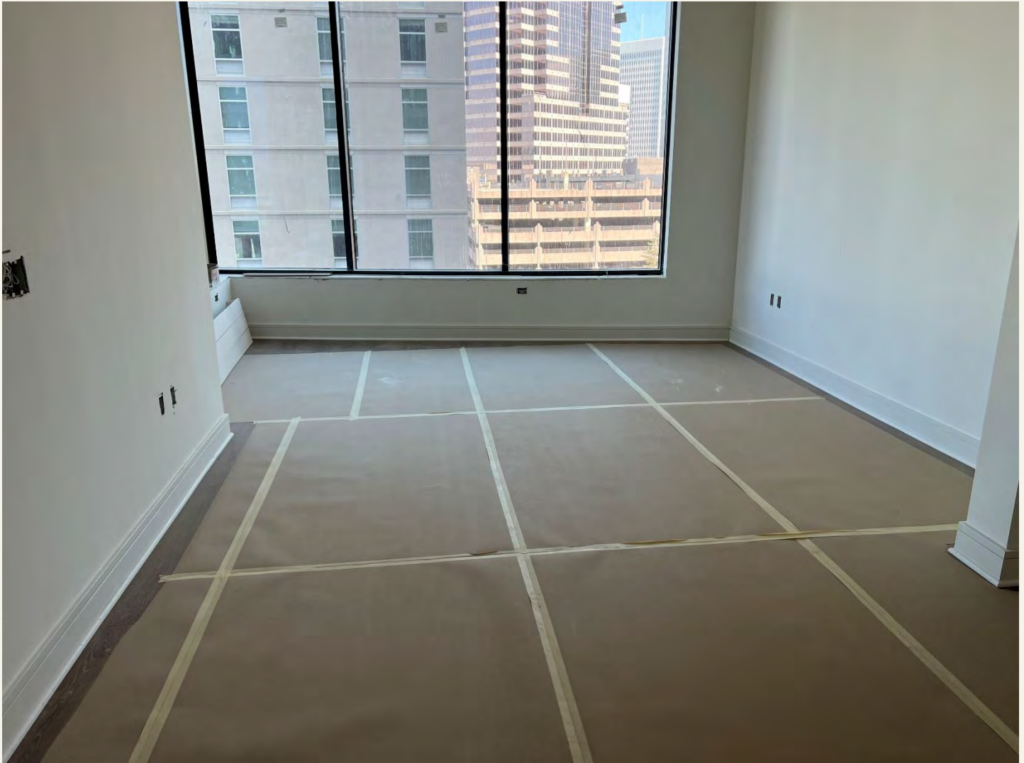
Description: Level 9 – Mockup Units Wood Flooring in Progress.
