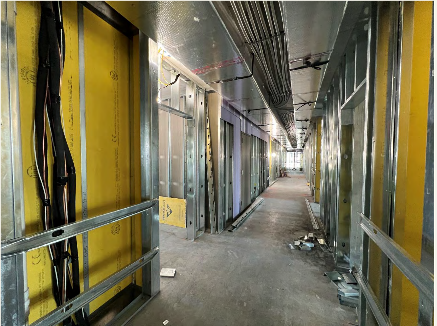
Description: Shaft Walls in Progress on Level 18.
