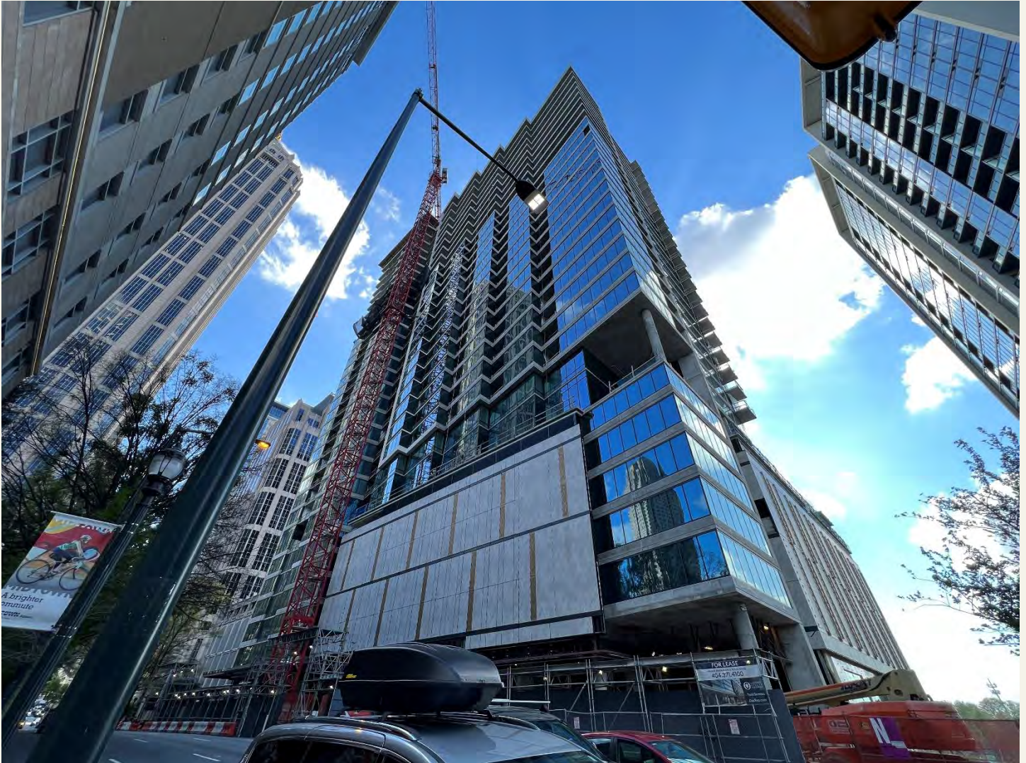
Description: Northeast Elevation of Site – Exterior Work in Progress.
