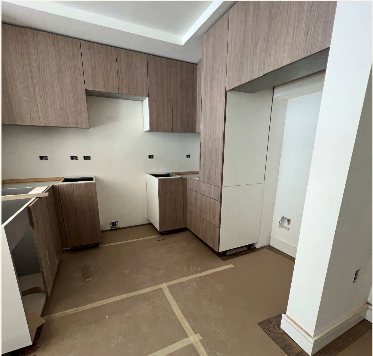
Description: Level 9 – Mockup Unit Kitchen Cabinets Installation in Progress.
