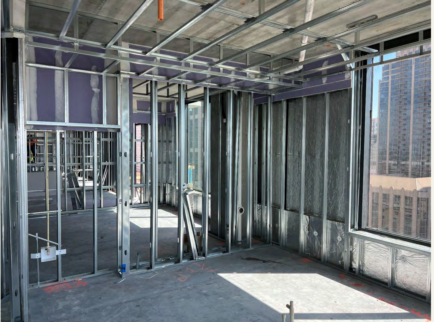
Description: Level 16 Perimeter Wall Insulation & Pre Rock Complete.
