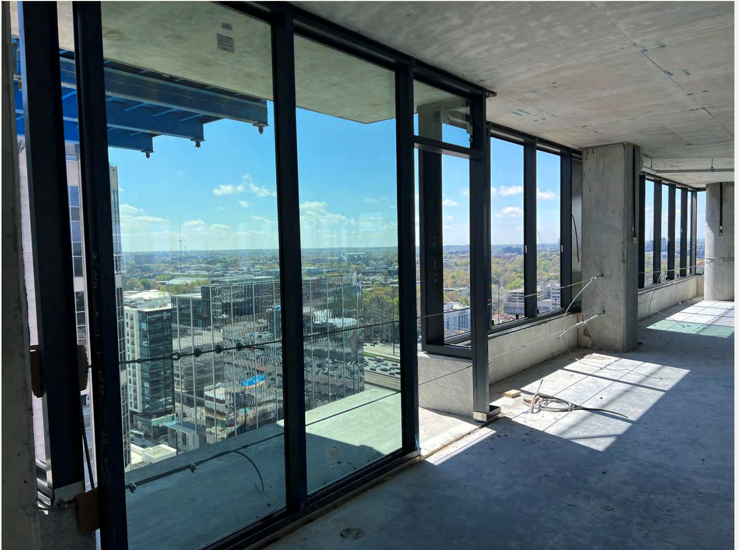
Description: Window Wall Glazing Installation in progress on Level 23.
