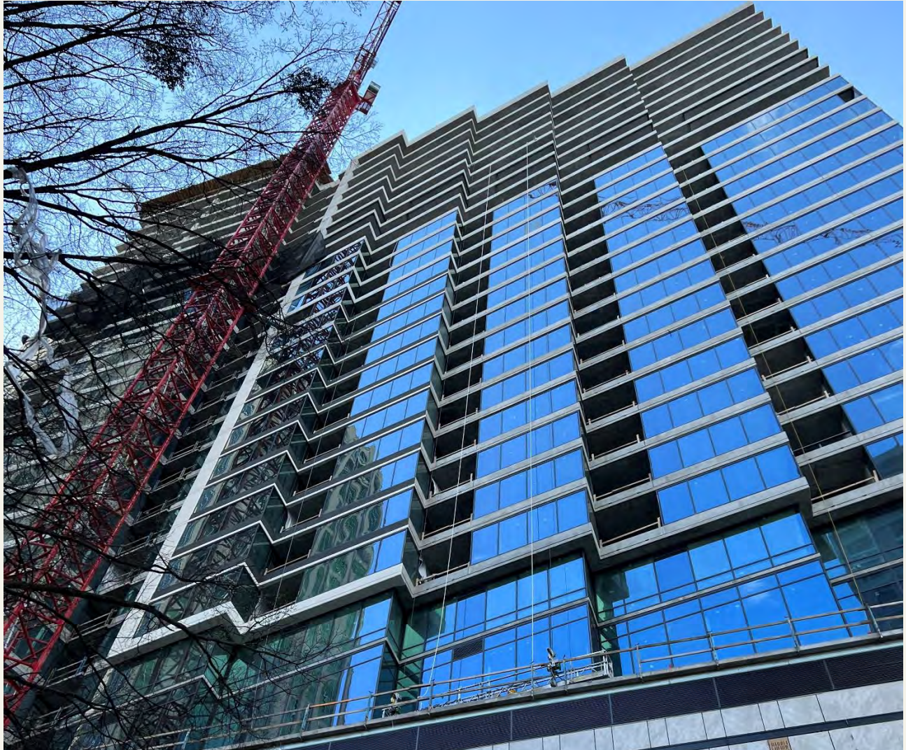
Description: Elastomeric Coating in Progress on East Elevation.
