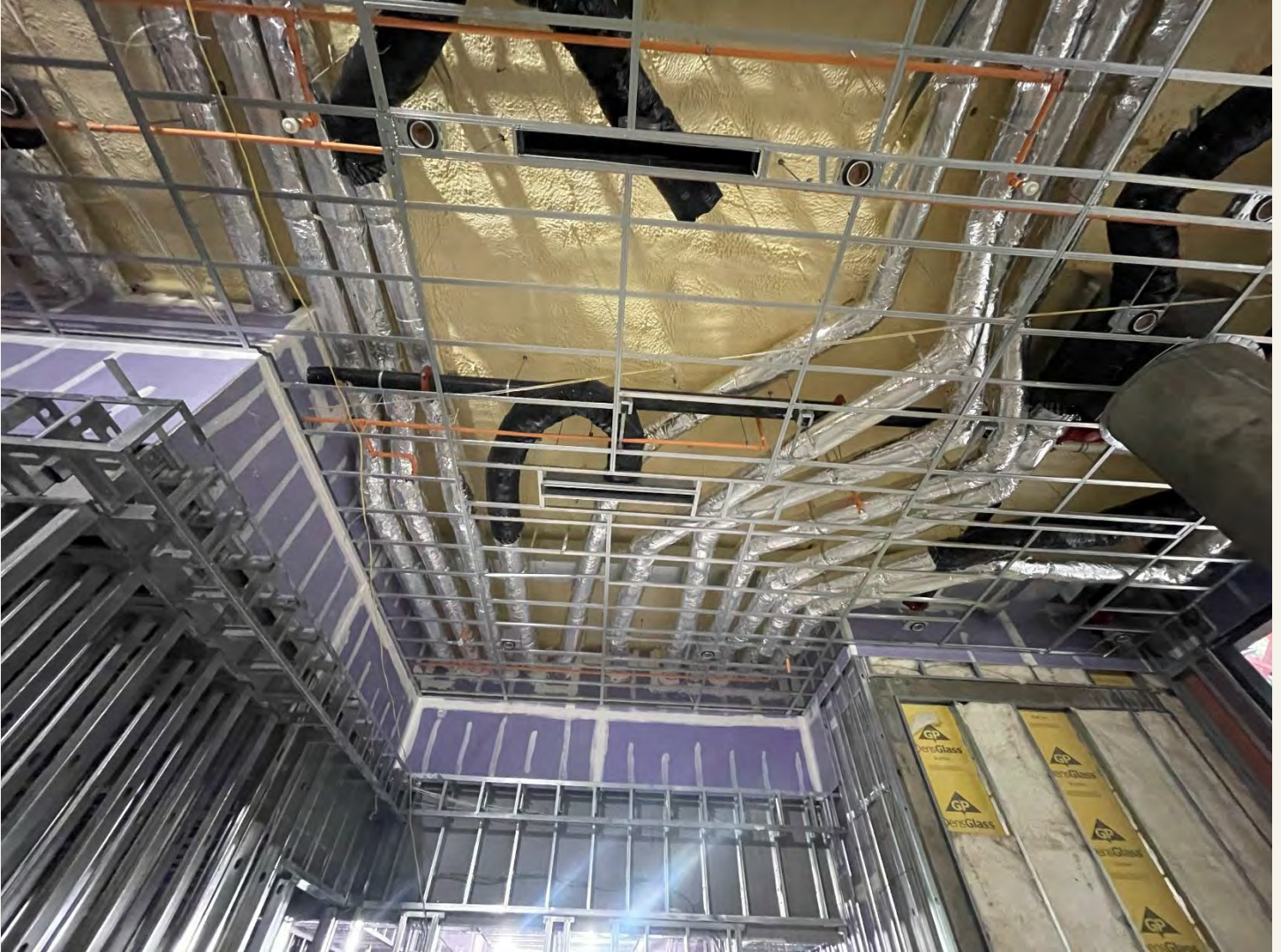
Description: Level 1 Lobby Design Team Box Walk Complete.
