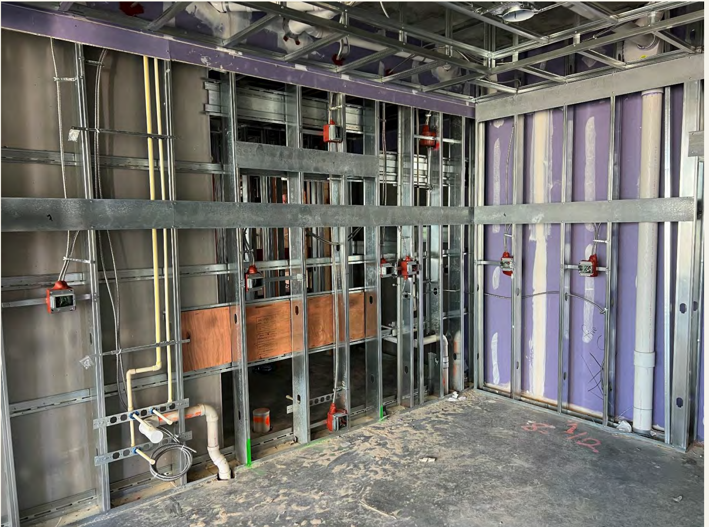
Description: Level 10 City Inspections in progress.
