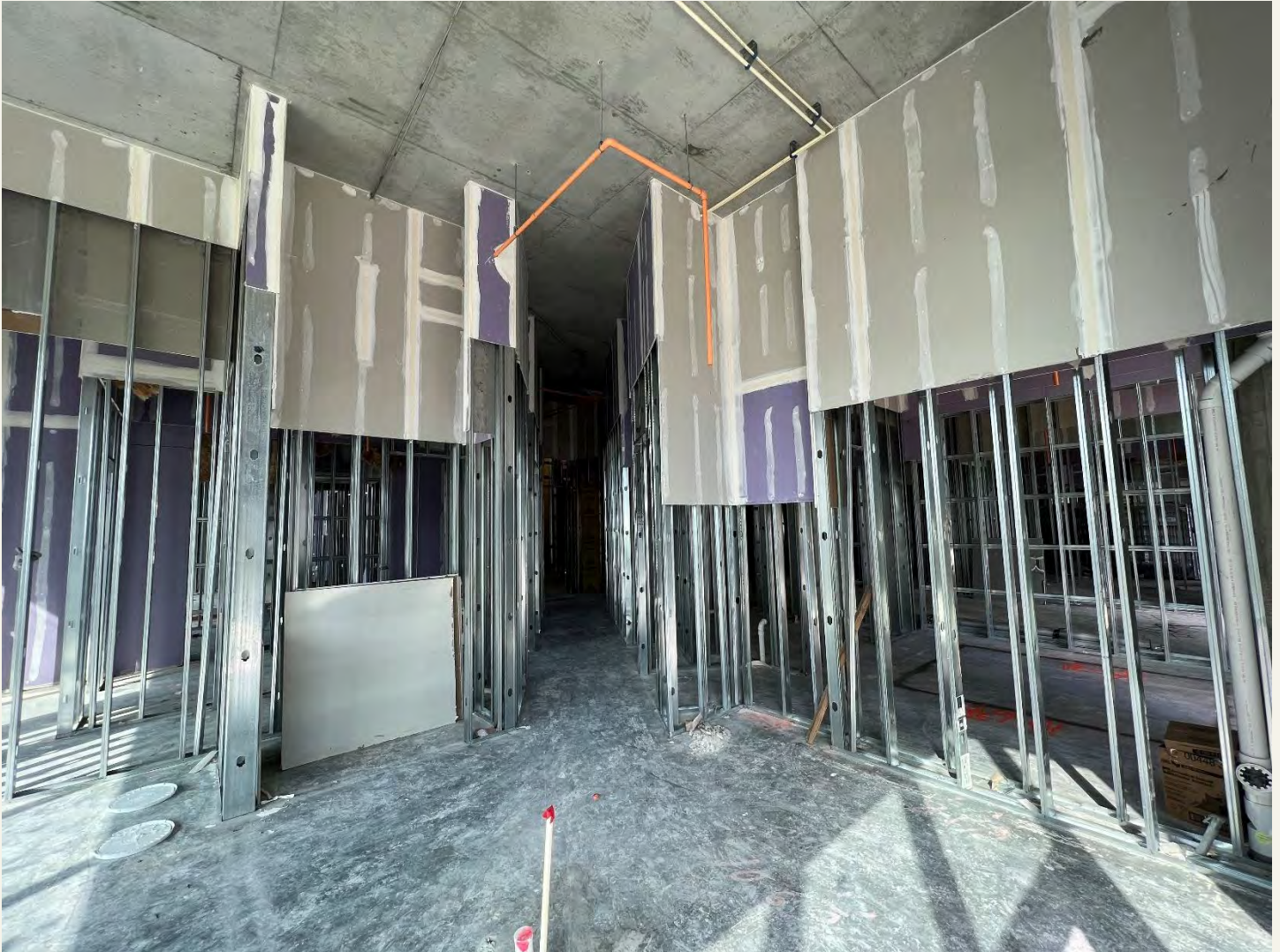
Description: Level 6 Amenity – Pre Rock in Progress.
