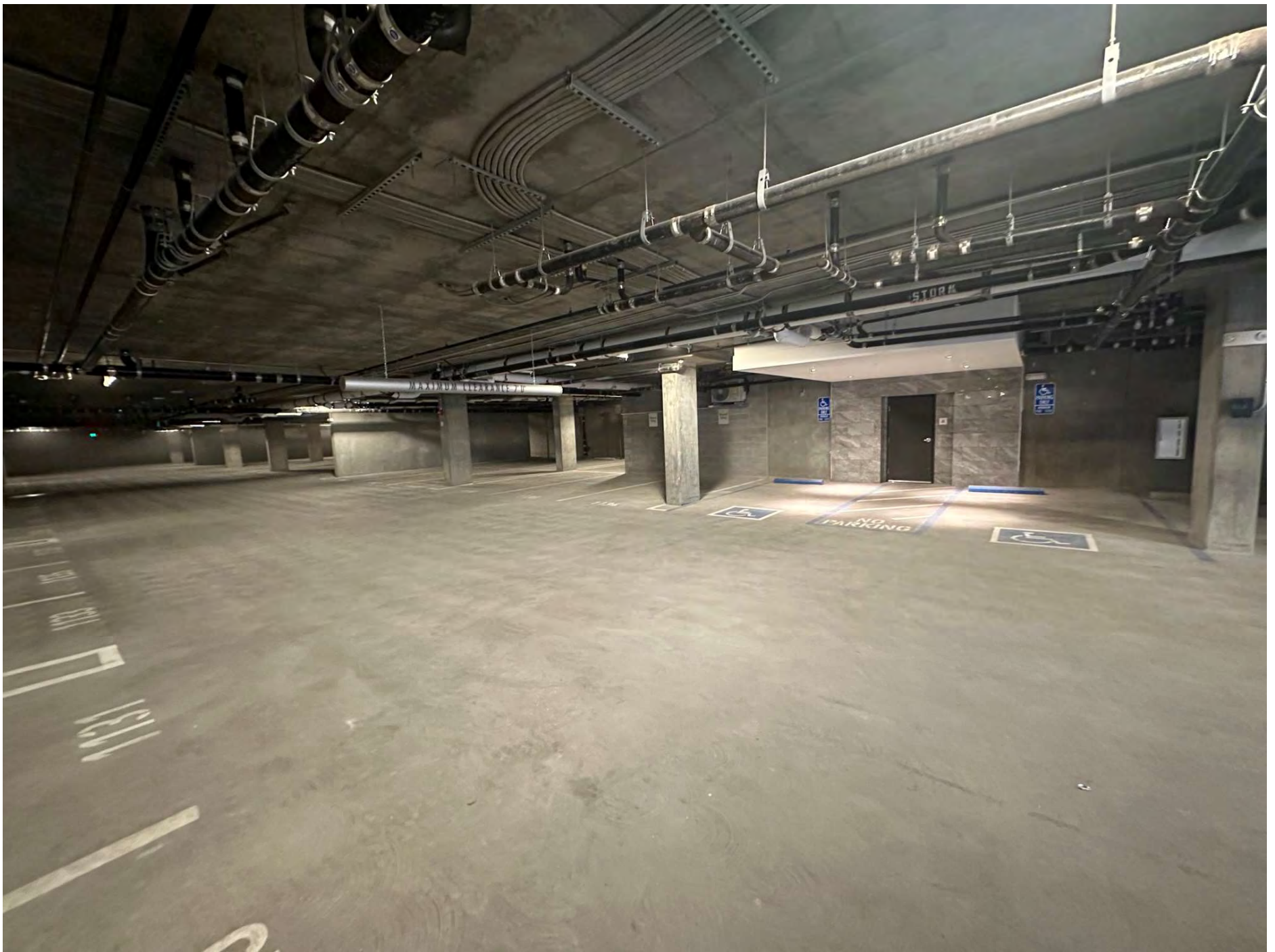
Garage: Building Inspection Near Complete
