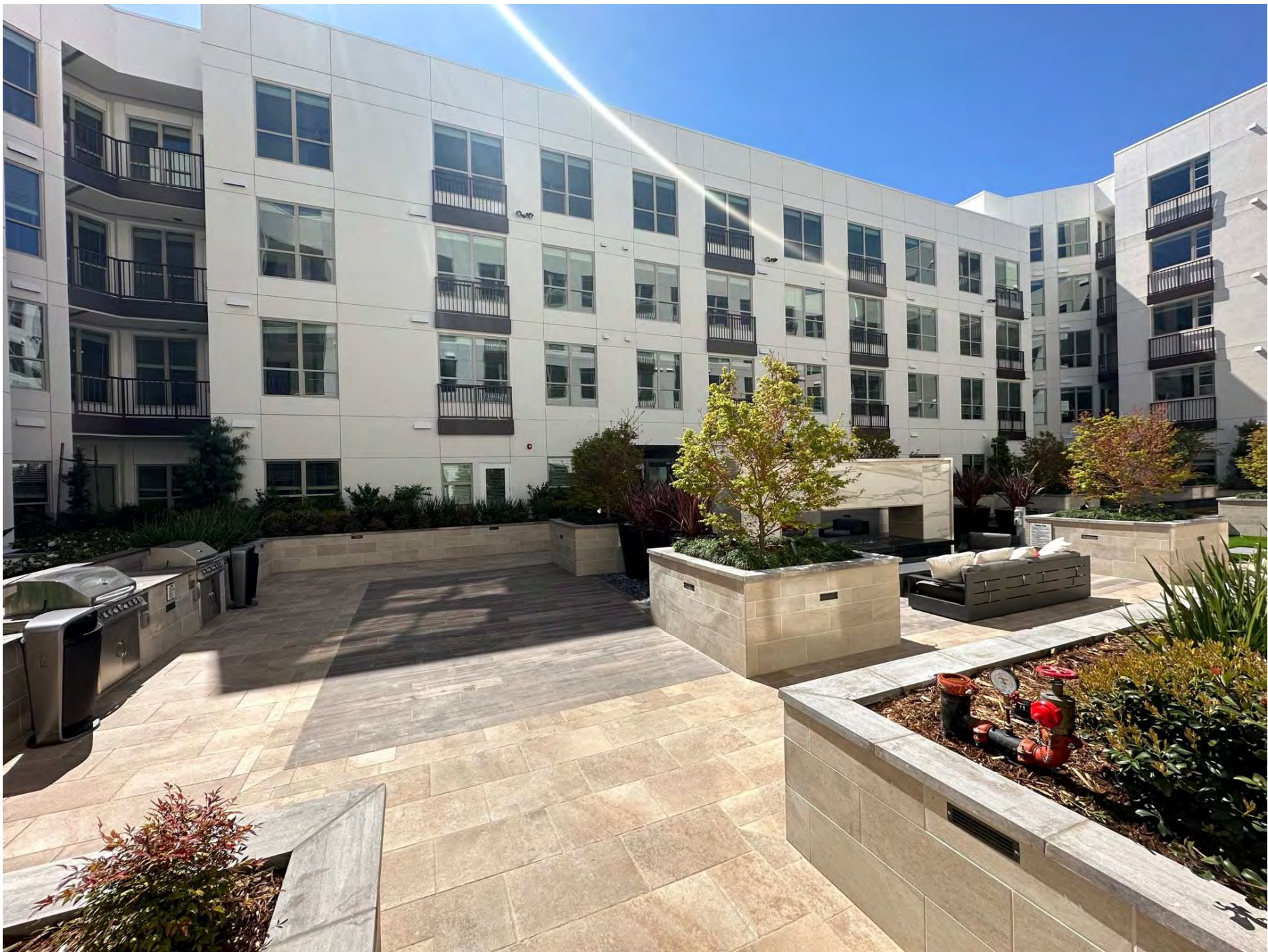
Courtyard B: Building Inspection Near Complete
