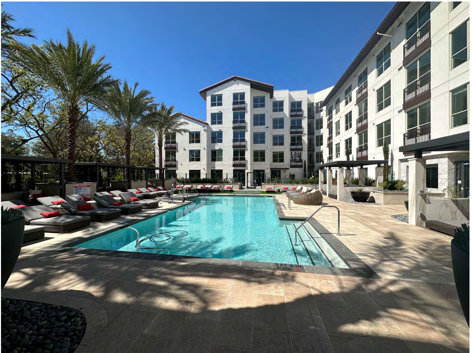
Courtyard A: Pool Final Inspection Complete
