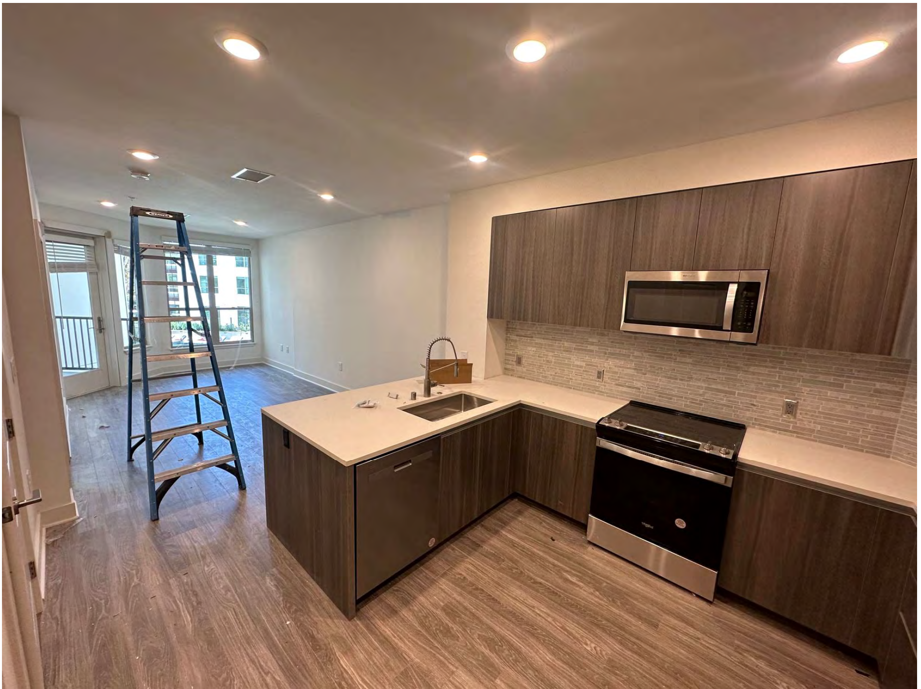
Level 3 Area 1: Hot Check & Construction Punch Ongoing
