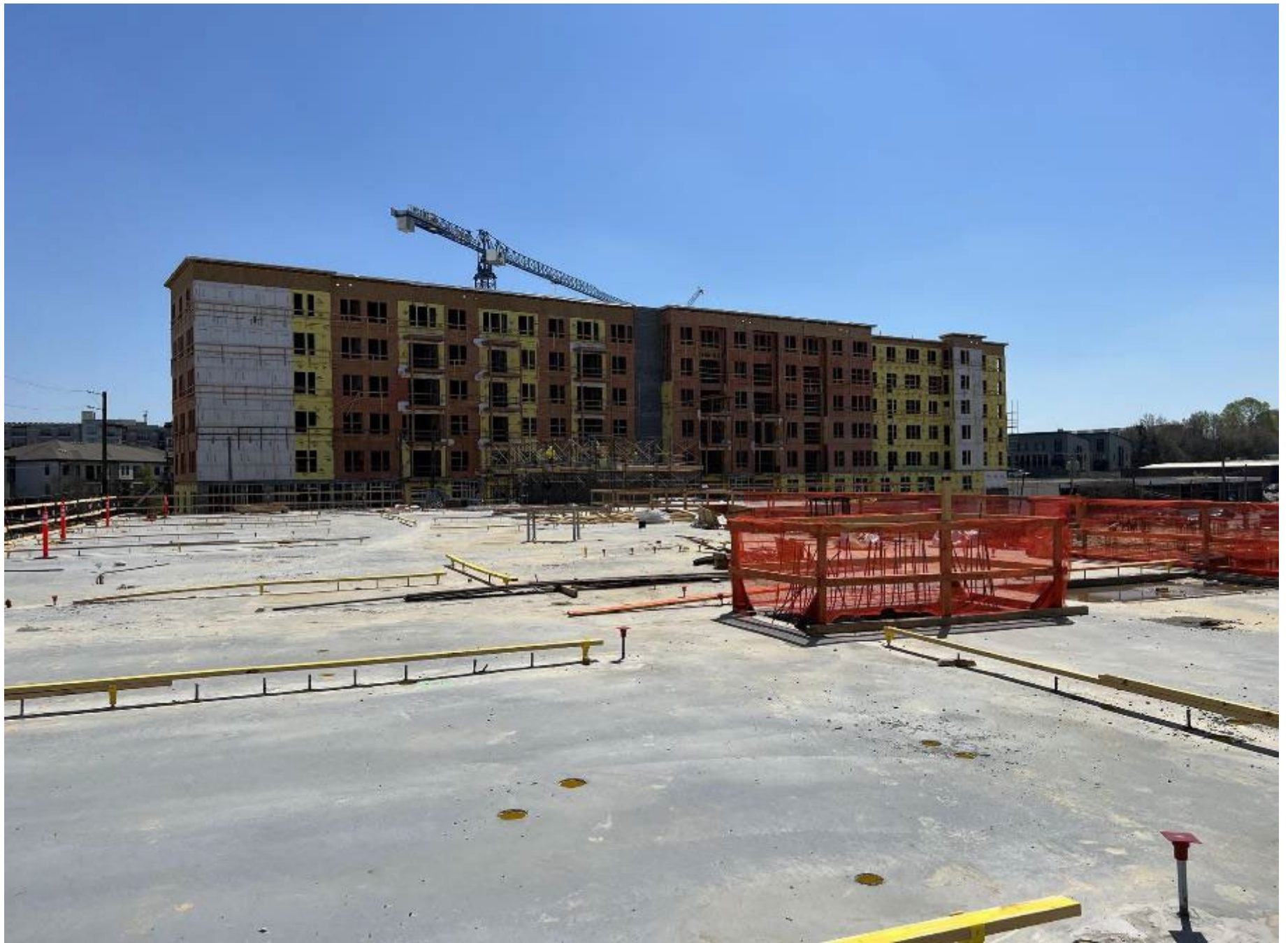
Photo Date: 3/24/23 Location: North viewing East
