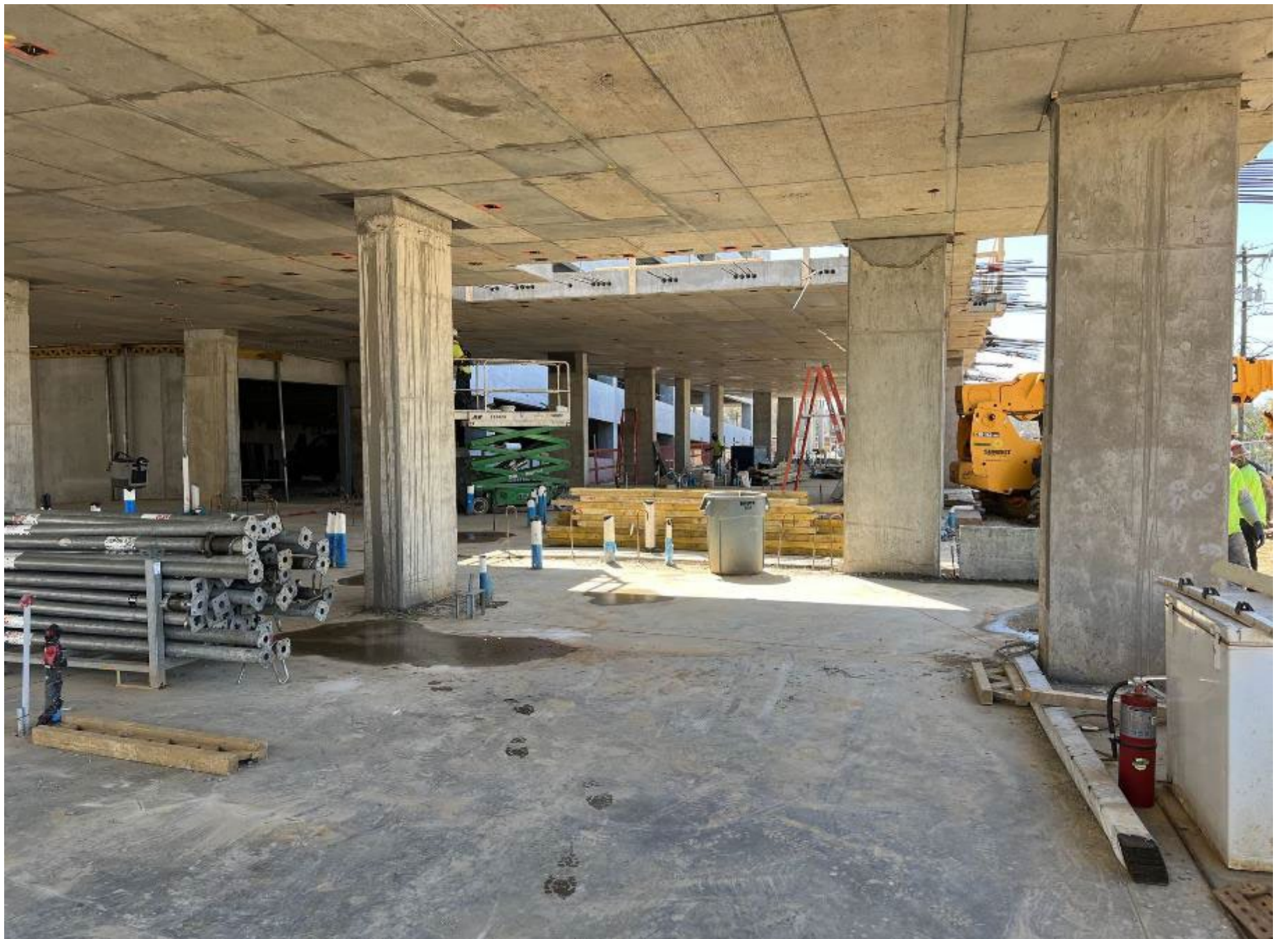
Photo Date: 3/24/23 Location: Northwest viewing South
