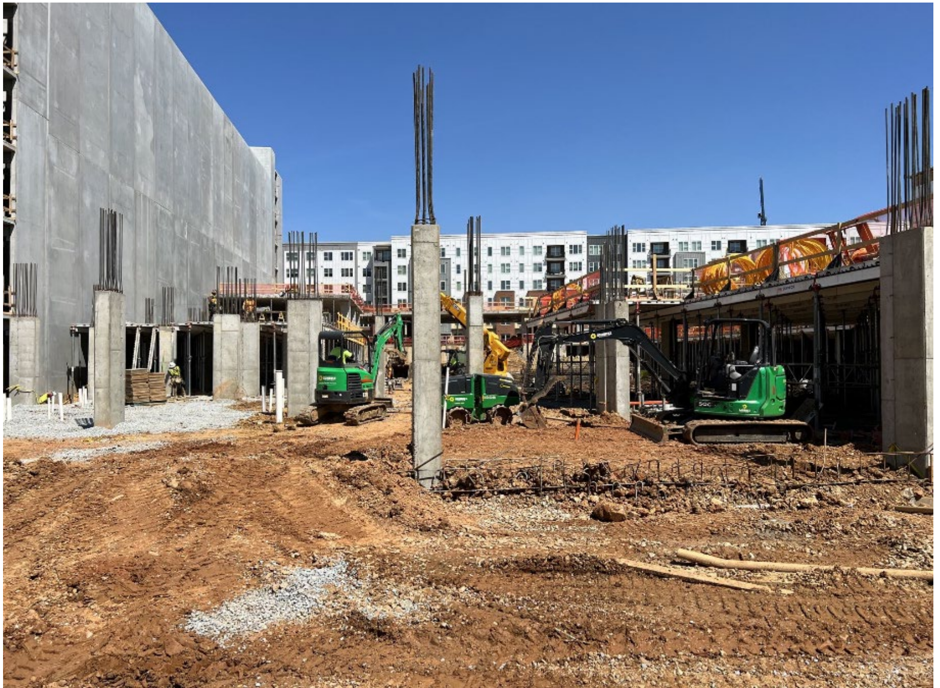
Photo Date: 3/24/23 Location: South viewing North
