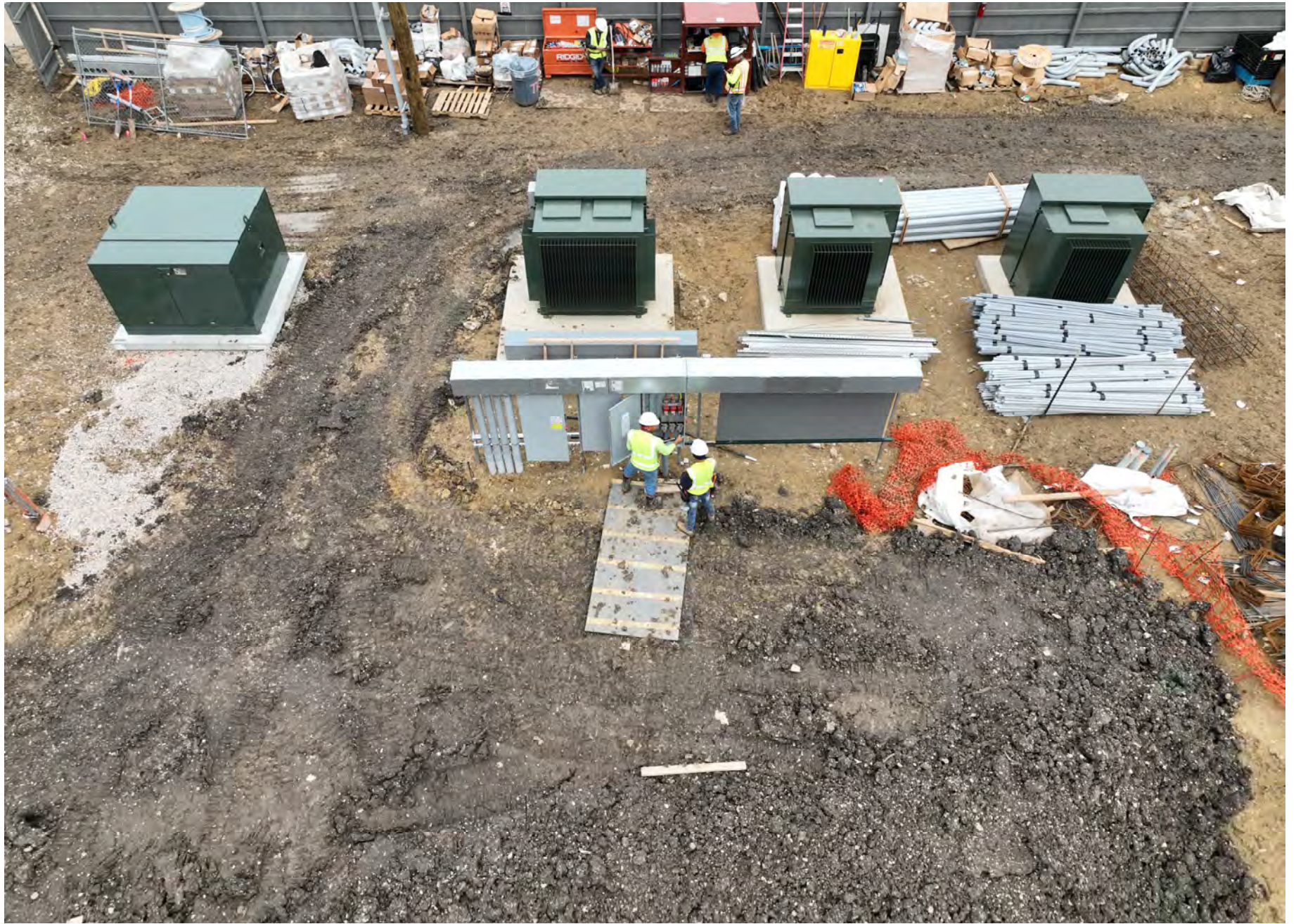
Temporary power distribution panel assembled, wire pulled to the tower crane.
