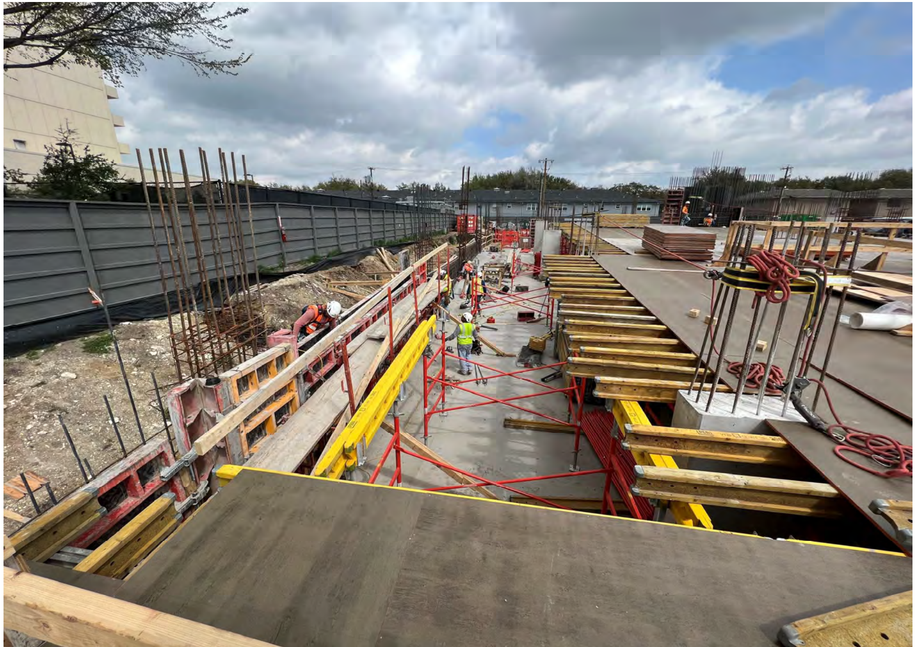
West retaining wall forming and placement continuing North.
