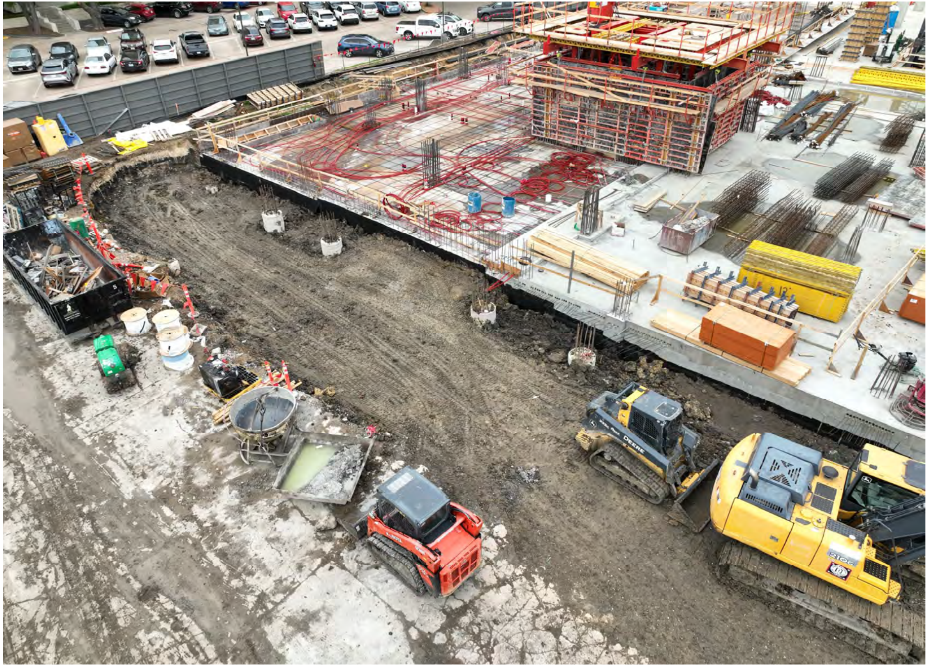
Below-grade waterproofing complete on South retaining wall, backfill to grade.
