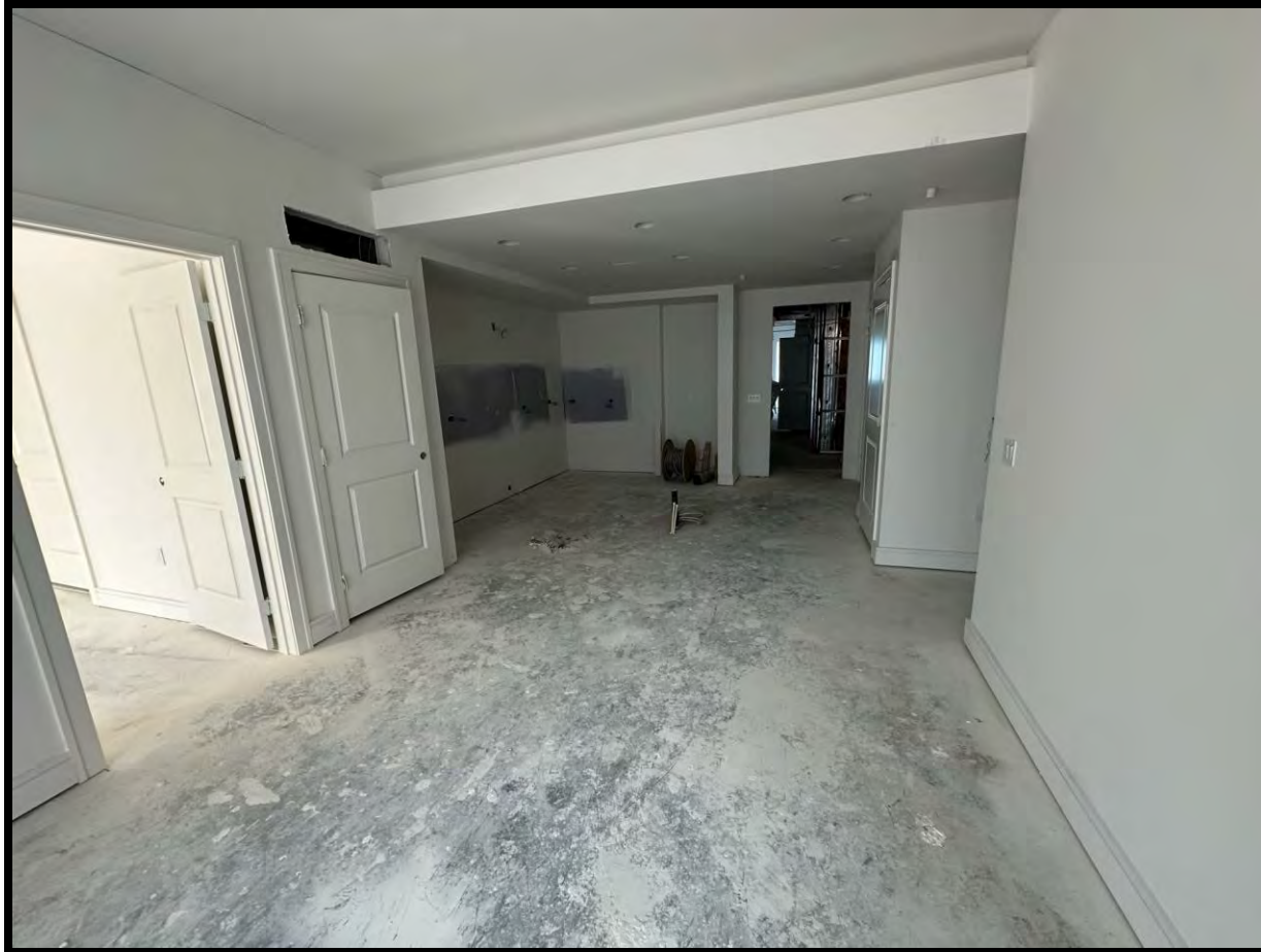
Photo Date: 03/24/2023 Location: Level 7 Units Description: Trim Installation is nearing completion
