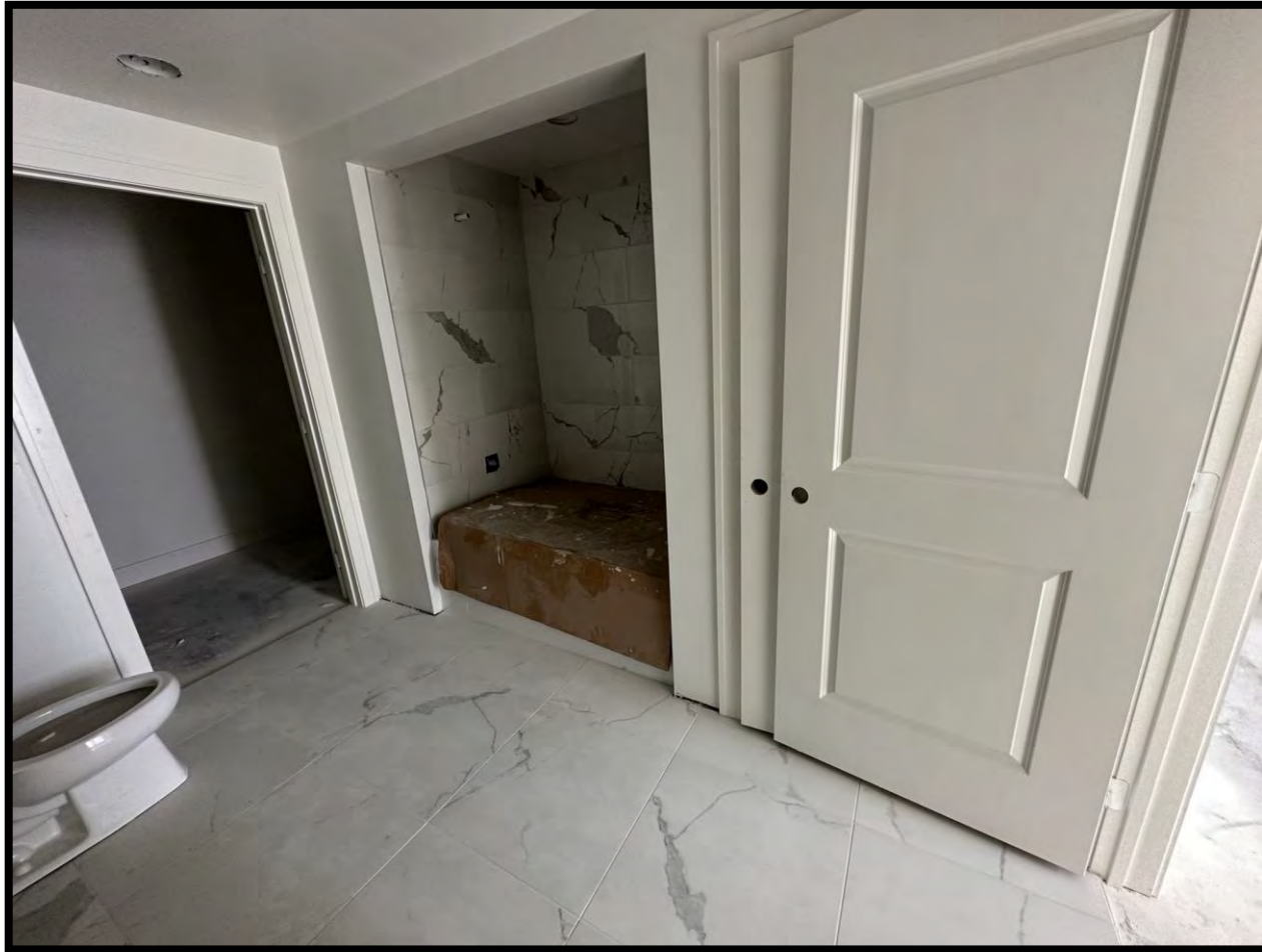
Photo Date: 03/24/2023 Location: Level 7 Units Description: Bathroom Tile install nearing completion.
