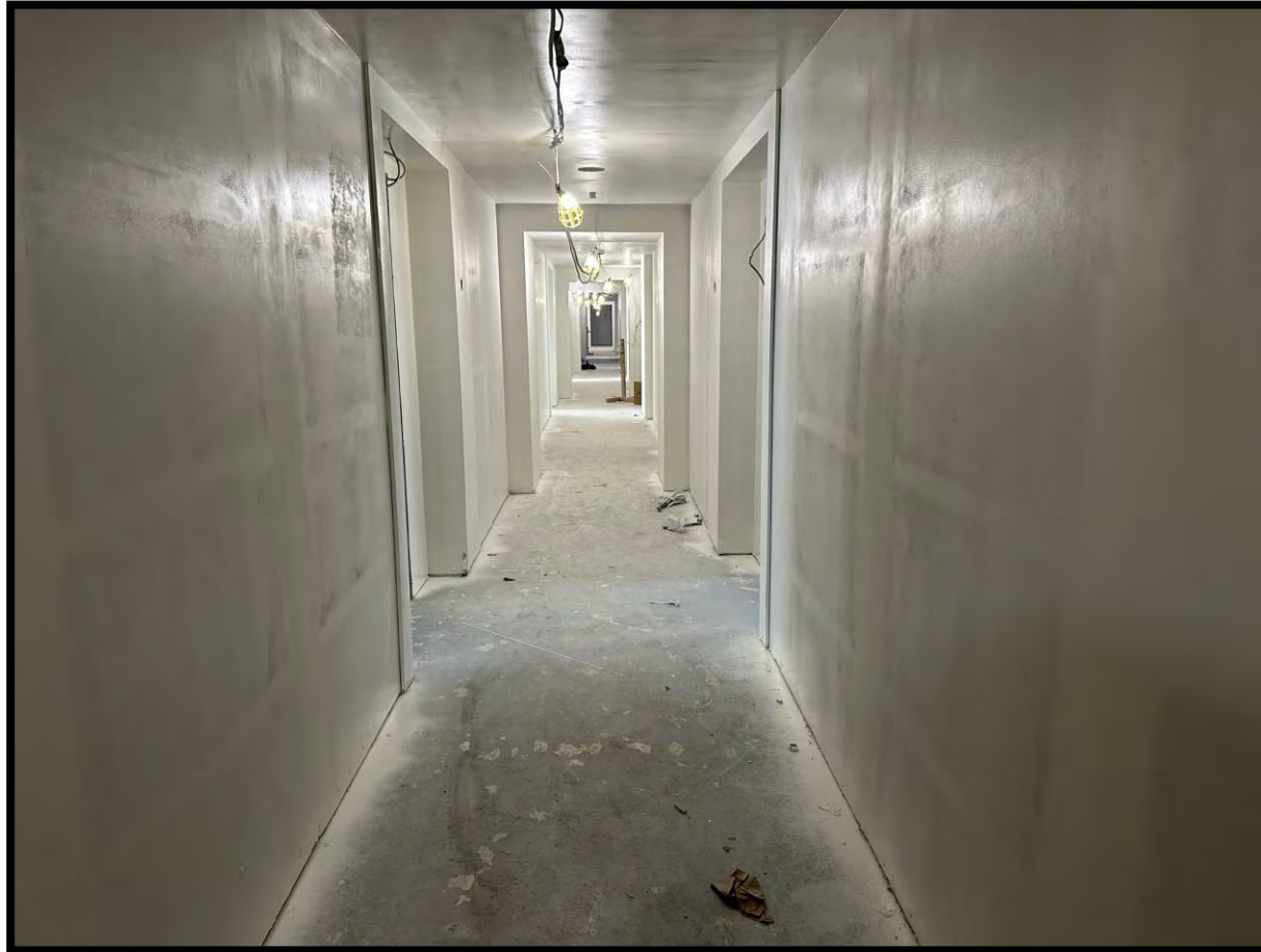
Photo Date: 03/24/2023 Location: Level 6 Corridor Description: Corridor Wall Priming is ongoing.
