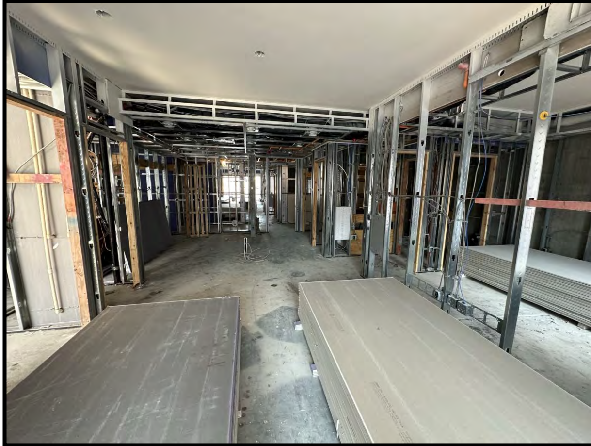
Photo Date: 03/24/2023 Location: Level 9 Units Description: MEP Inspections are ongoing.
