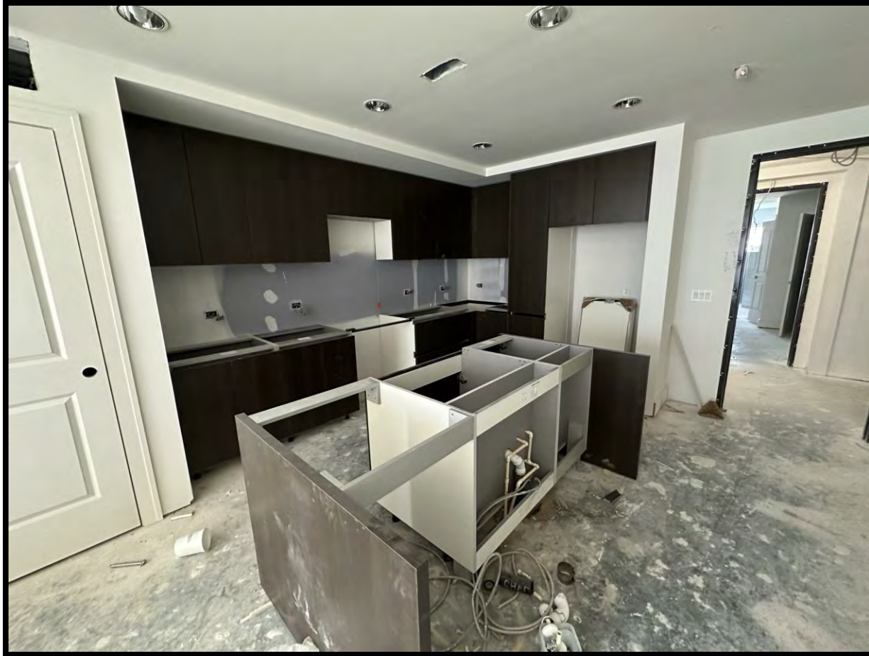
Photo Date: 03/24/2023 Location: Level 6 Units Description: Cabinets installation is ongoing
