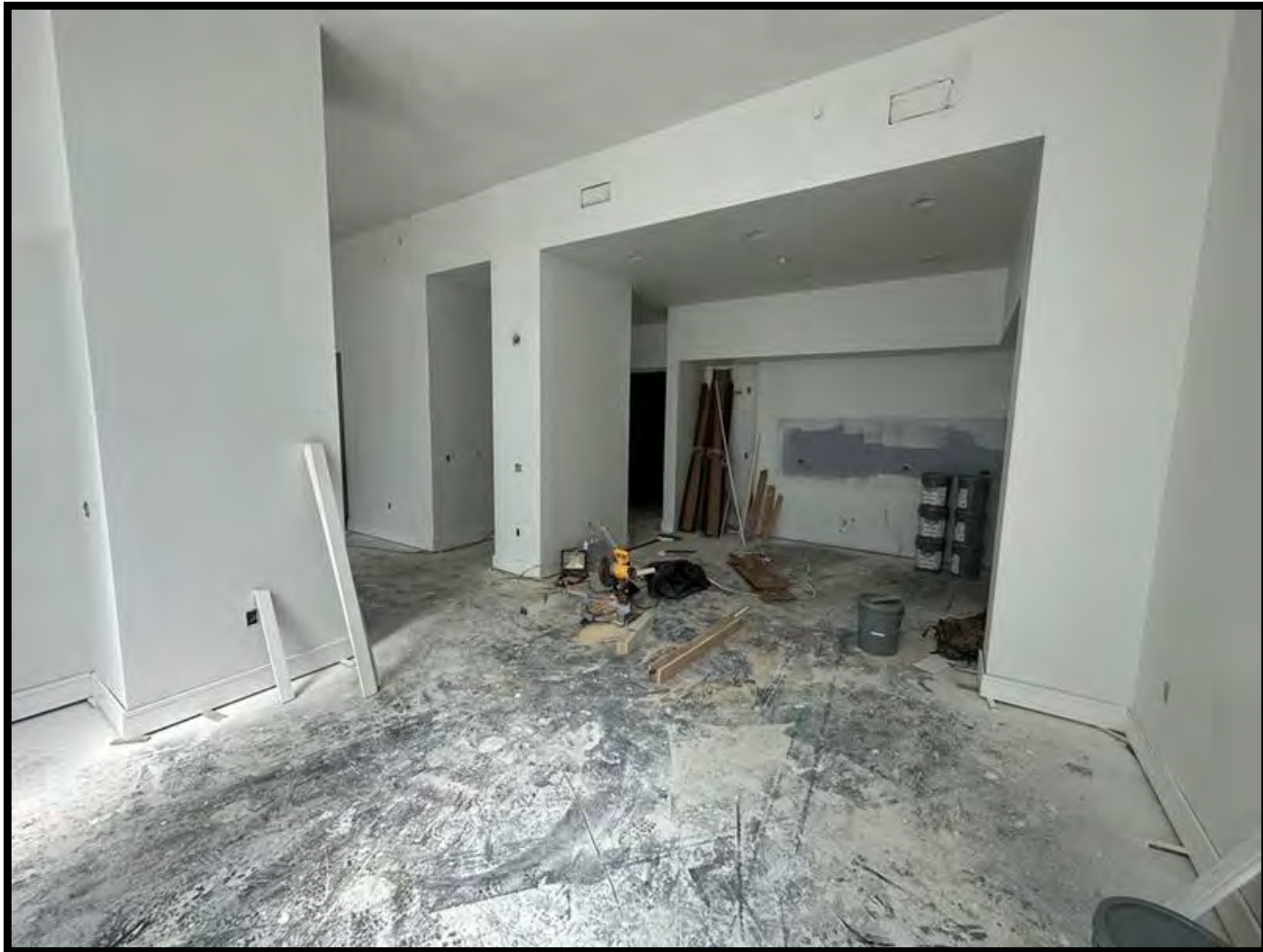
Photo Date: 03/24/2023 Location: Townhome Units Description: Trim Installation is ongoing.
