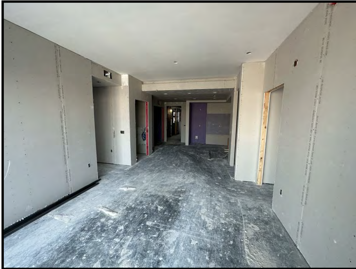
Photo Date: 03/24/2023 Location: Level 8 Units Description: Drywall is ongoing.
