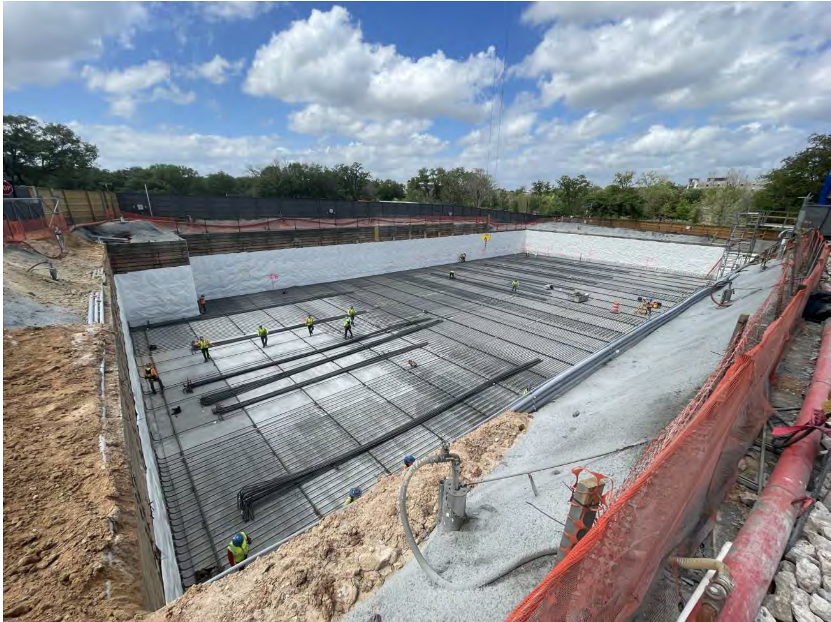
3/22/2023: Mat foundation reinforcement progress
