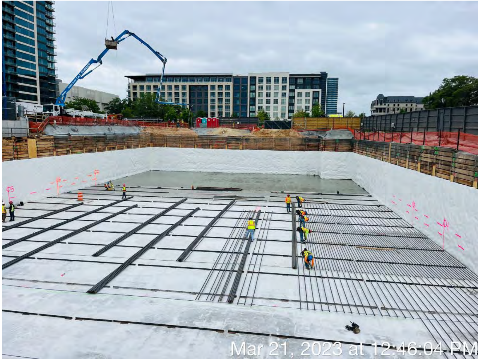
03/21/2023: Start of reinforcement for mat foundation
