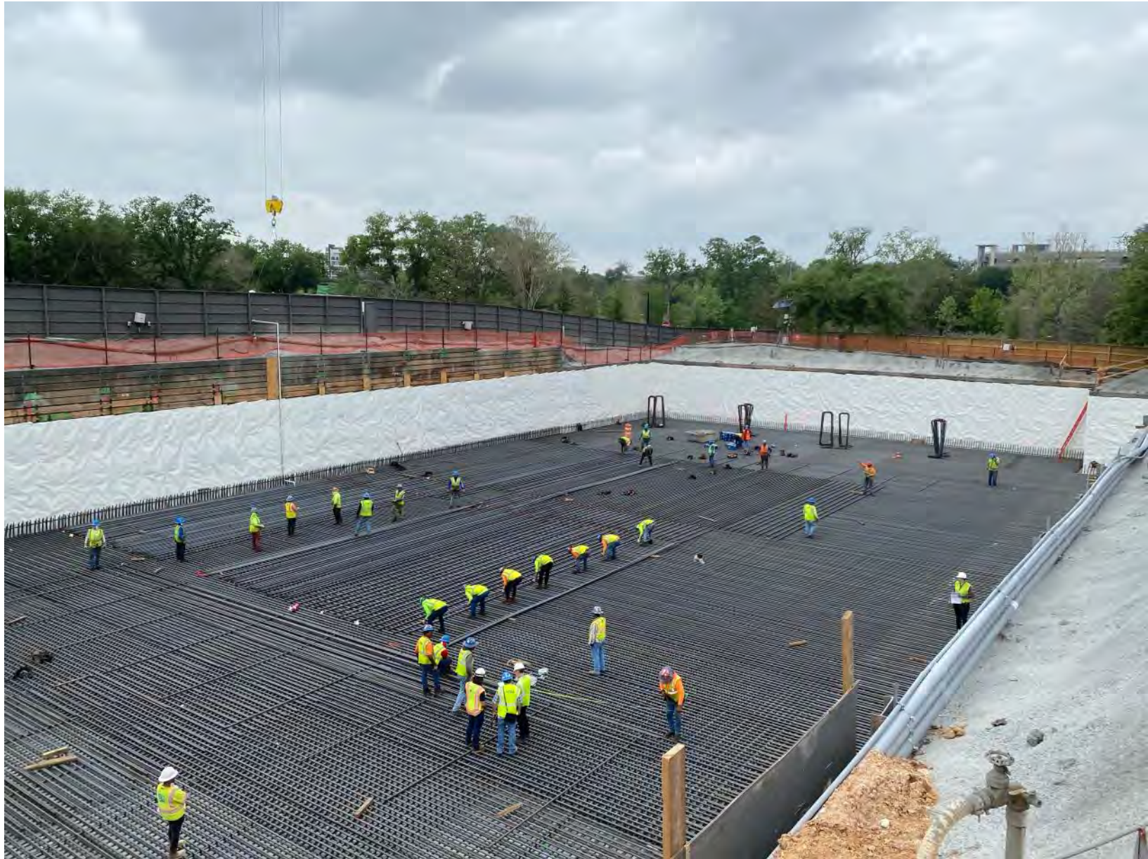
02/24/2023: SCA (structural engineer) onsite to review bottom of mat reinforcement
