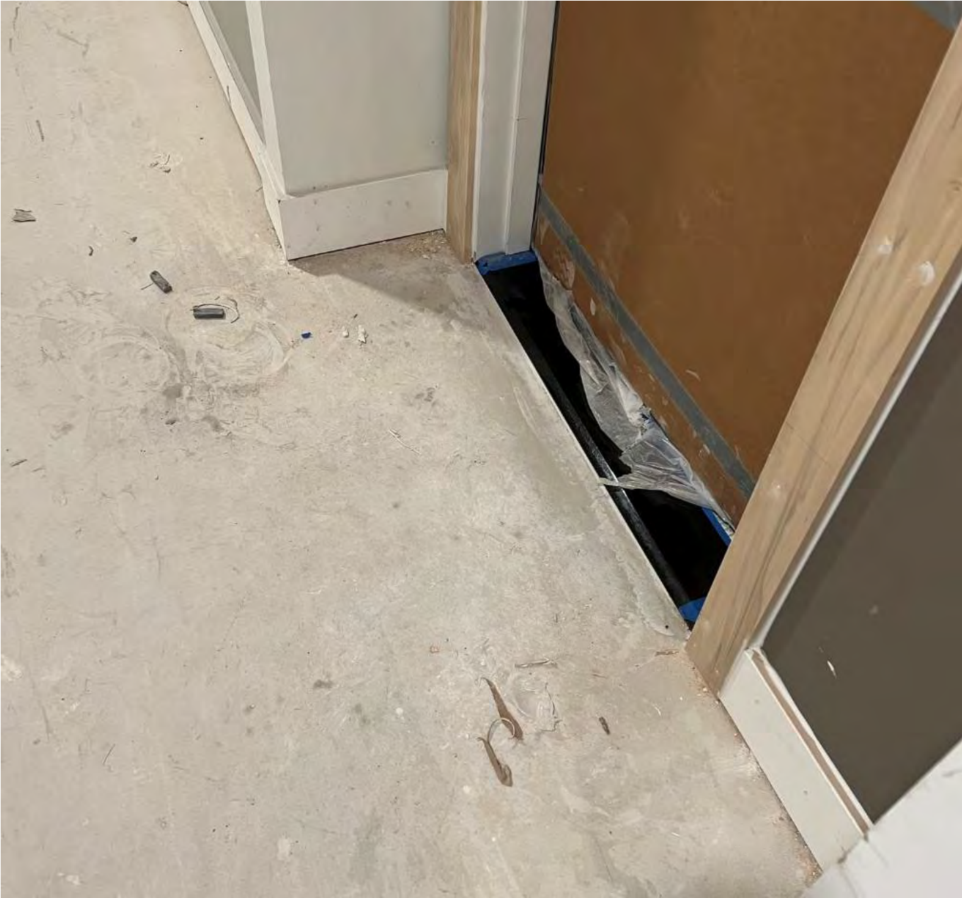
Phase 1, Level 5, Thresholds Installation Ongoing
