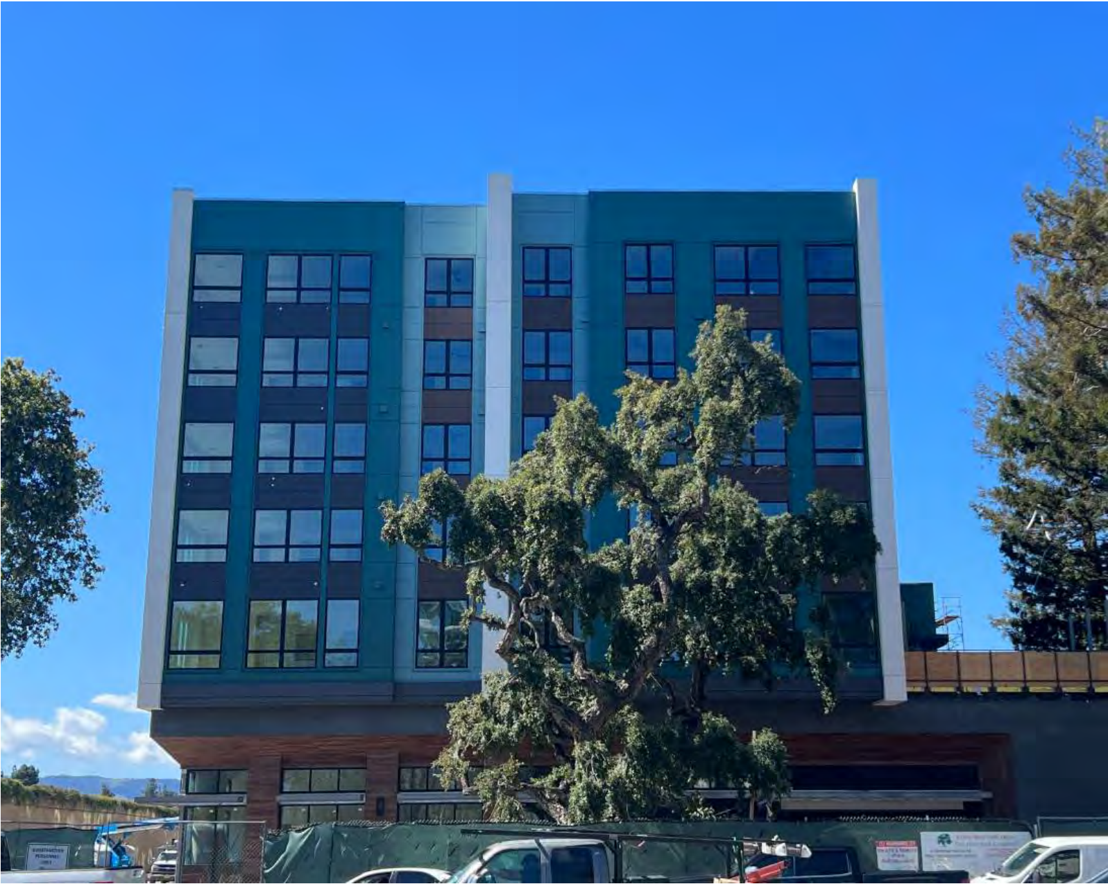
View of East Elevation
