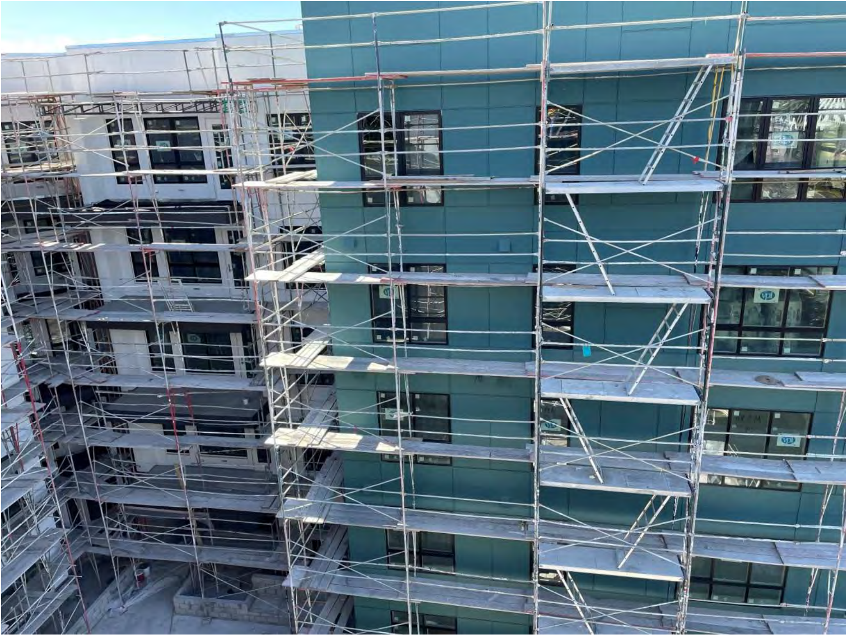
Aerial View of Courtyard C – West Elevation
