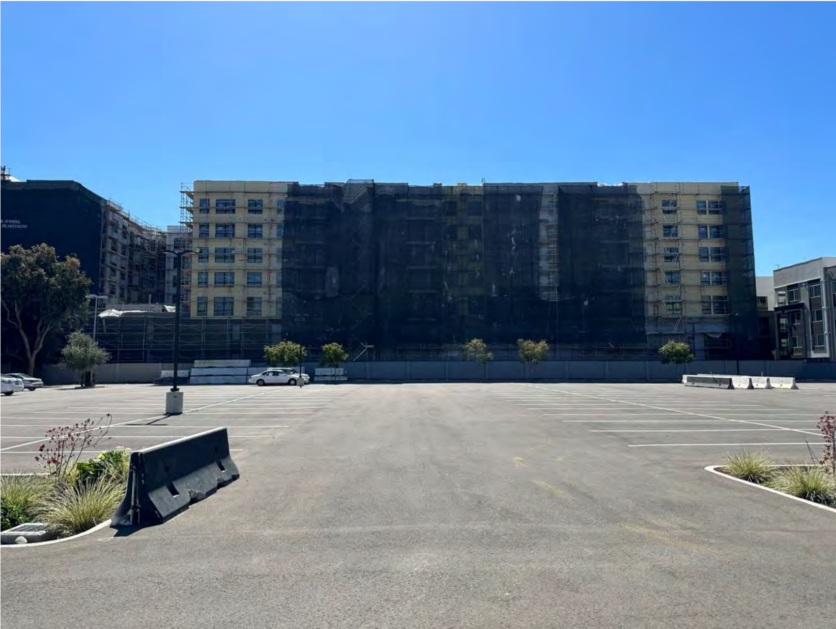
View of North Elevation
