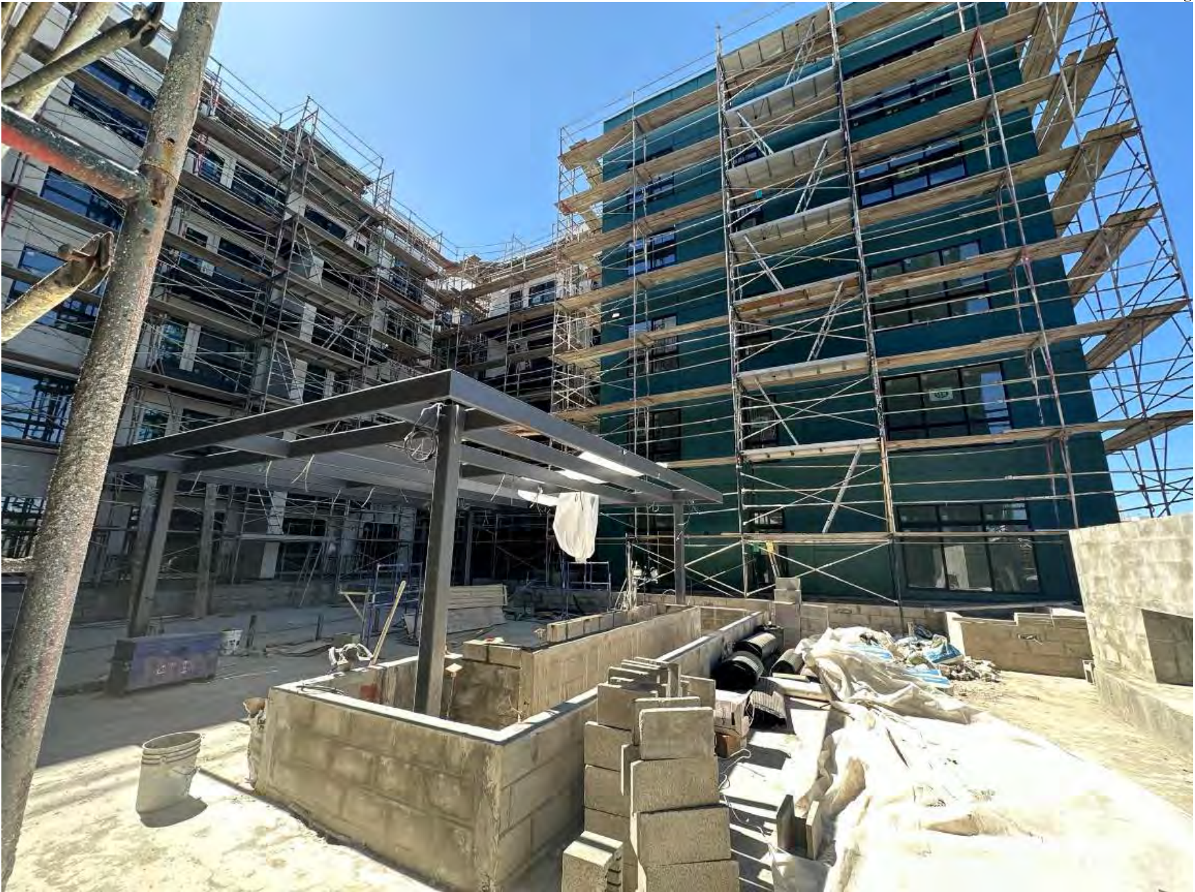
Ground View of Courtyard C
