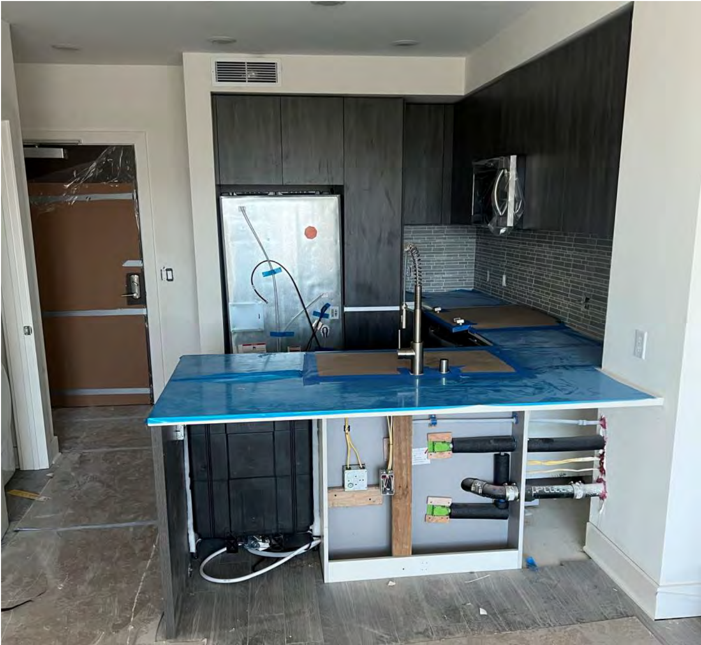
Phase 1, Level 6 - Unit MEP Trim Pick Up and Appliance Install Ongoing
