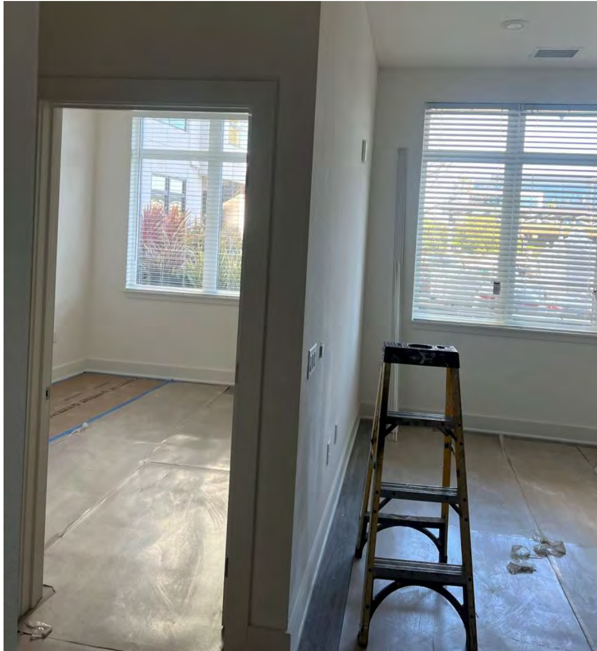
Phase 1, Level 3 - QAQC Ongoing
