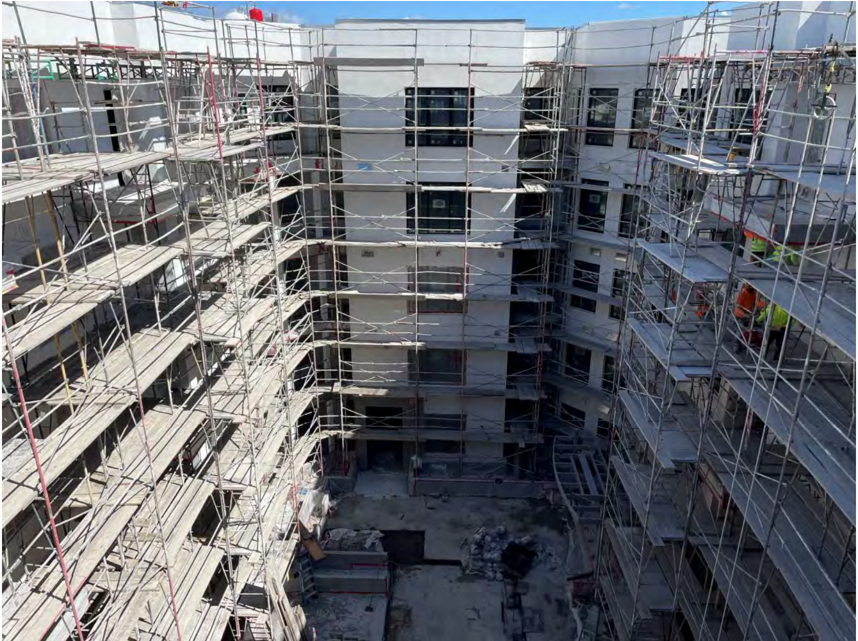
Aerial View of Courtyard D
