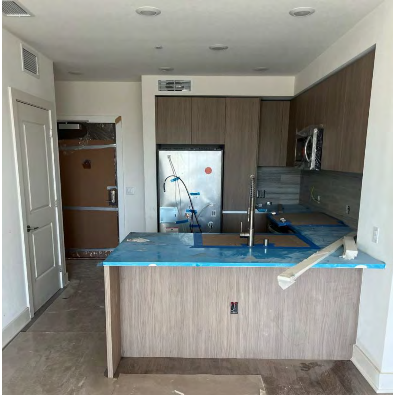
Phase 1, Level 5, Unit MEP Pick Up Ongoing
