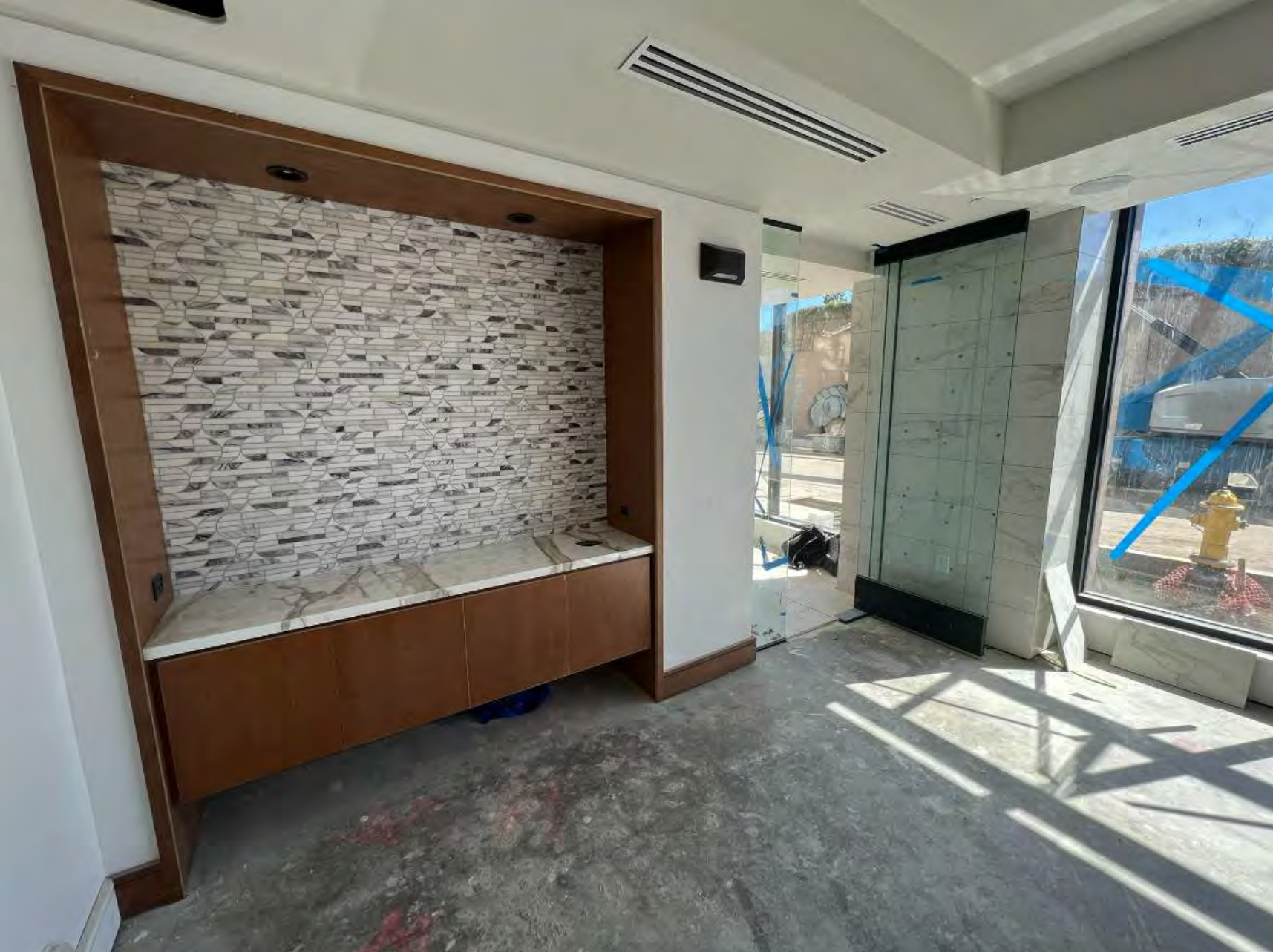
Phase 1, Level 1 – Meeting Room
