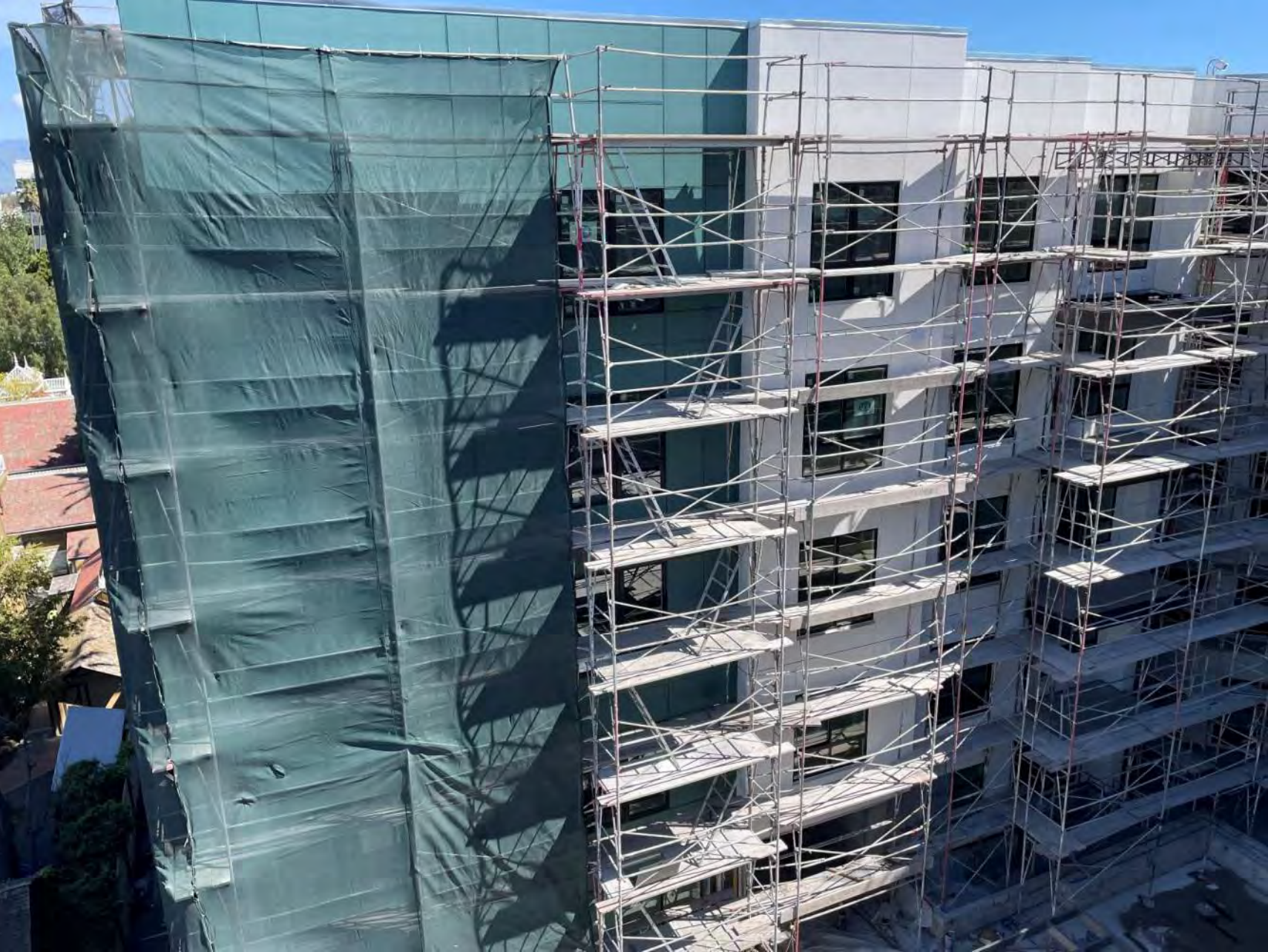
Aerial View of Courtyard C – East Elevation
