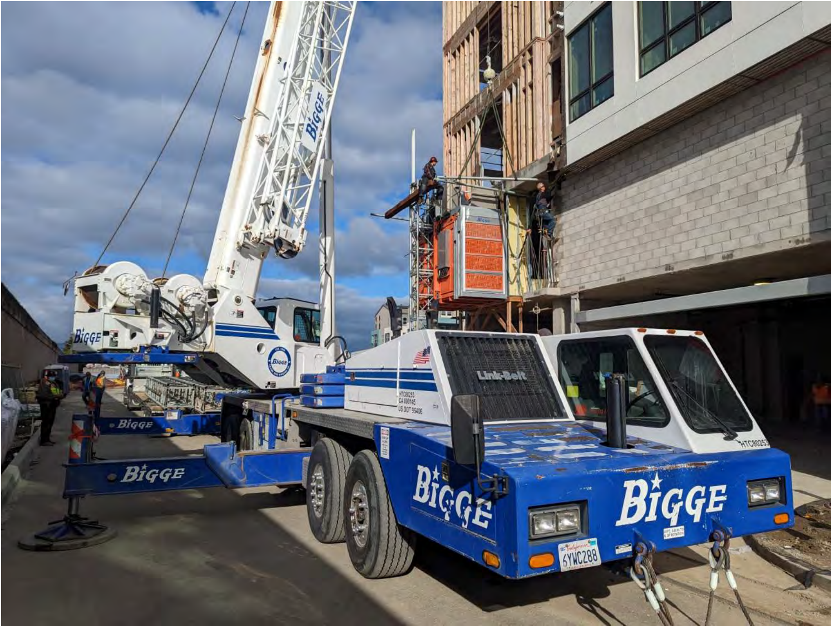
Personnel Hoist Demobilization
