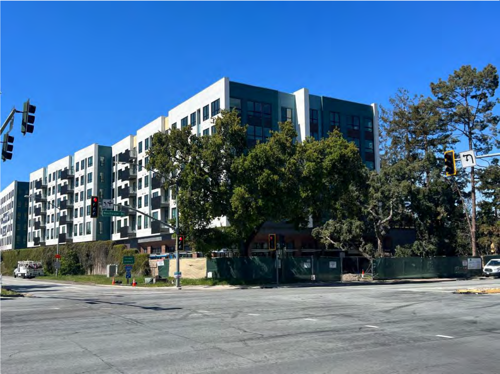
View of Southeast Elevation
