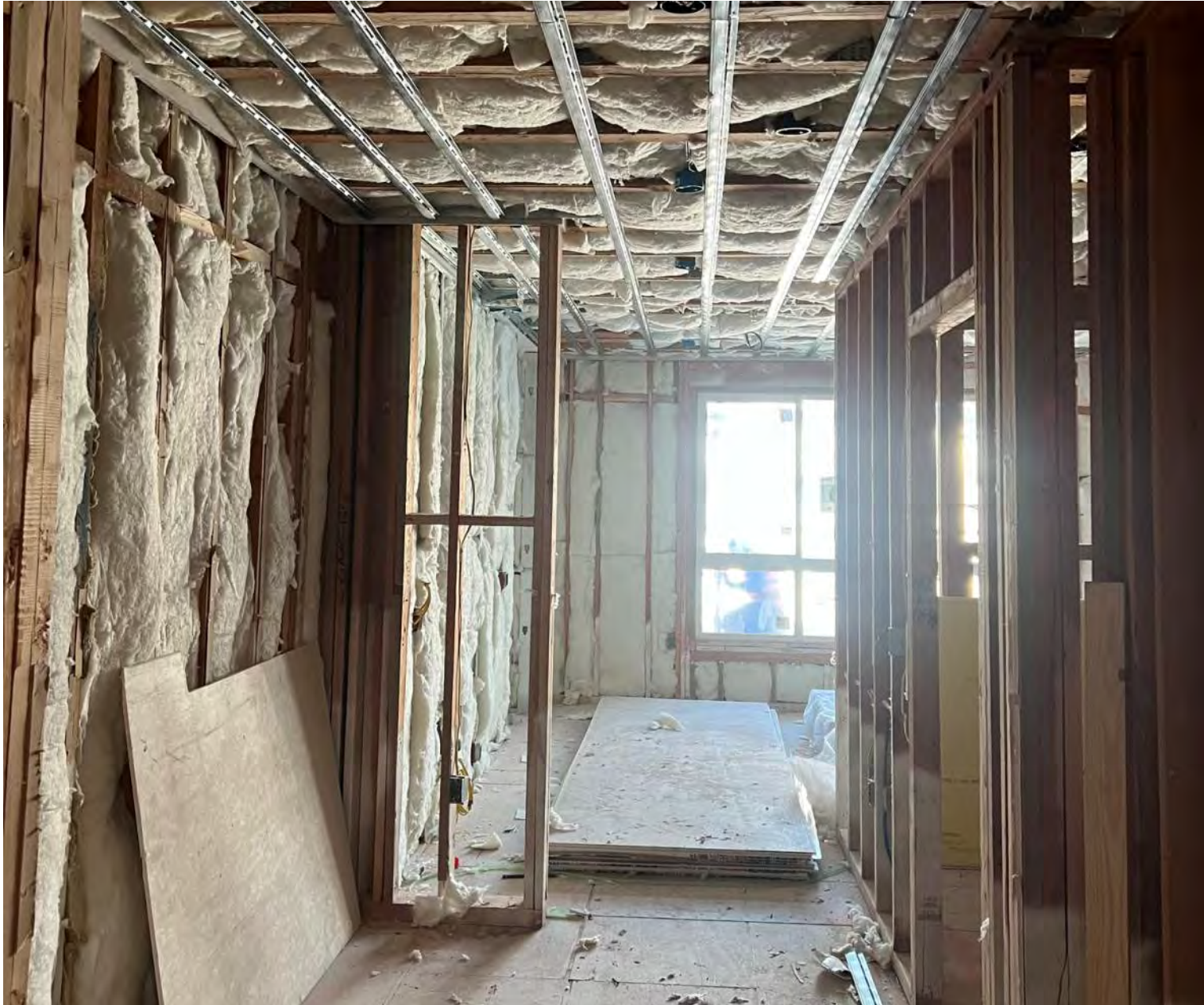
Phase 2, Level 6 – Insulation and RC Production Ongoing
