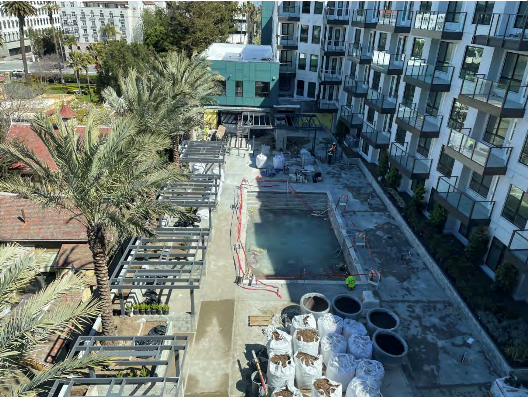
Aerial View of Courtyard B
