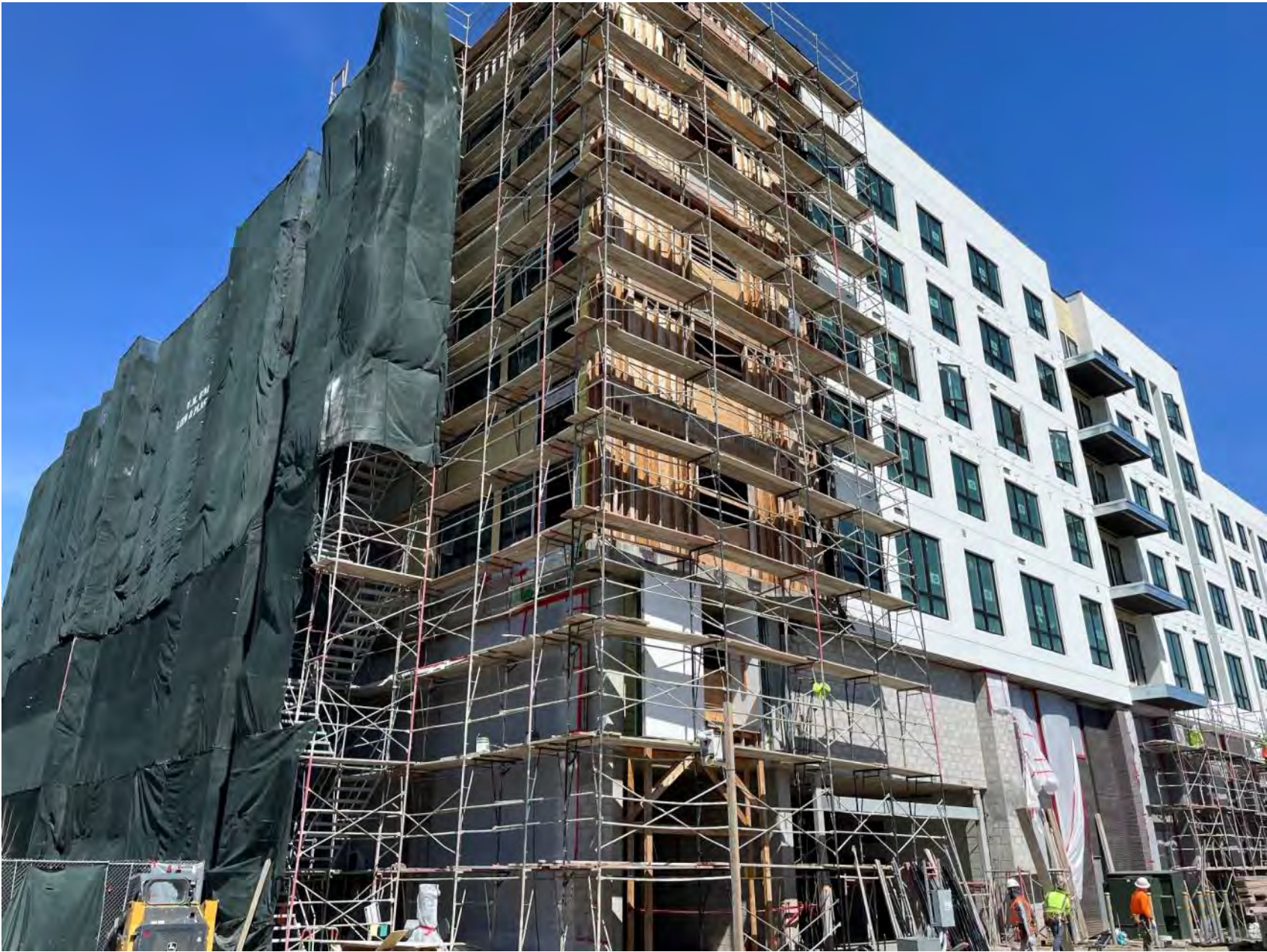
View of Southwest Elevation
