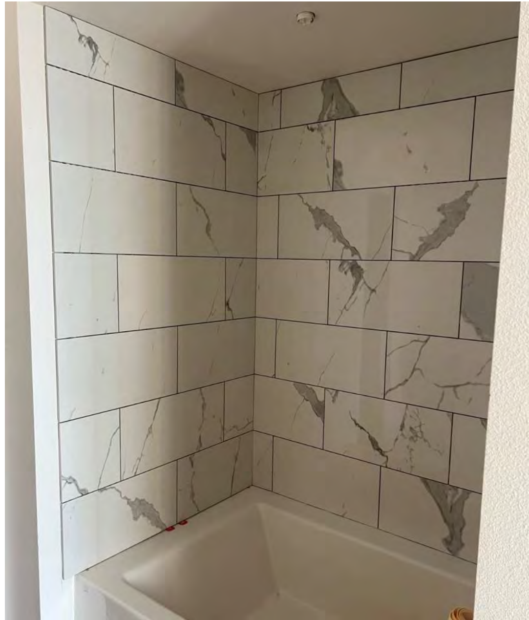
Phase 2, Level 4 – Unit Bathroom Tile Installation Ongoing
