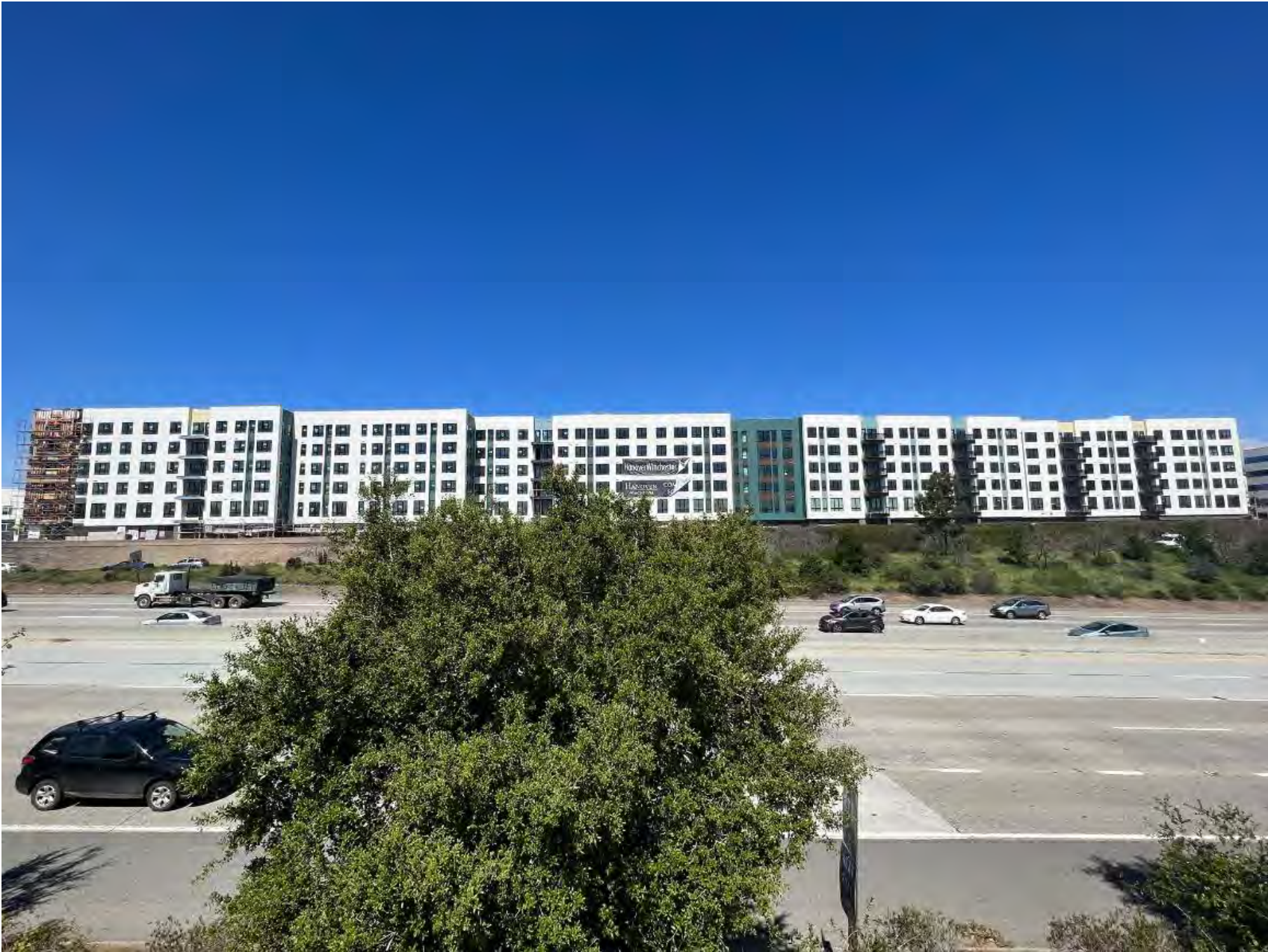
View of Southern Elevation
