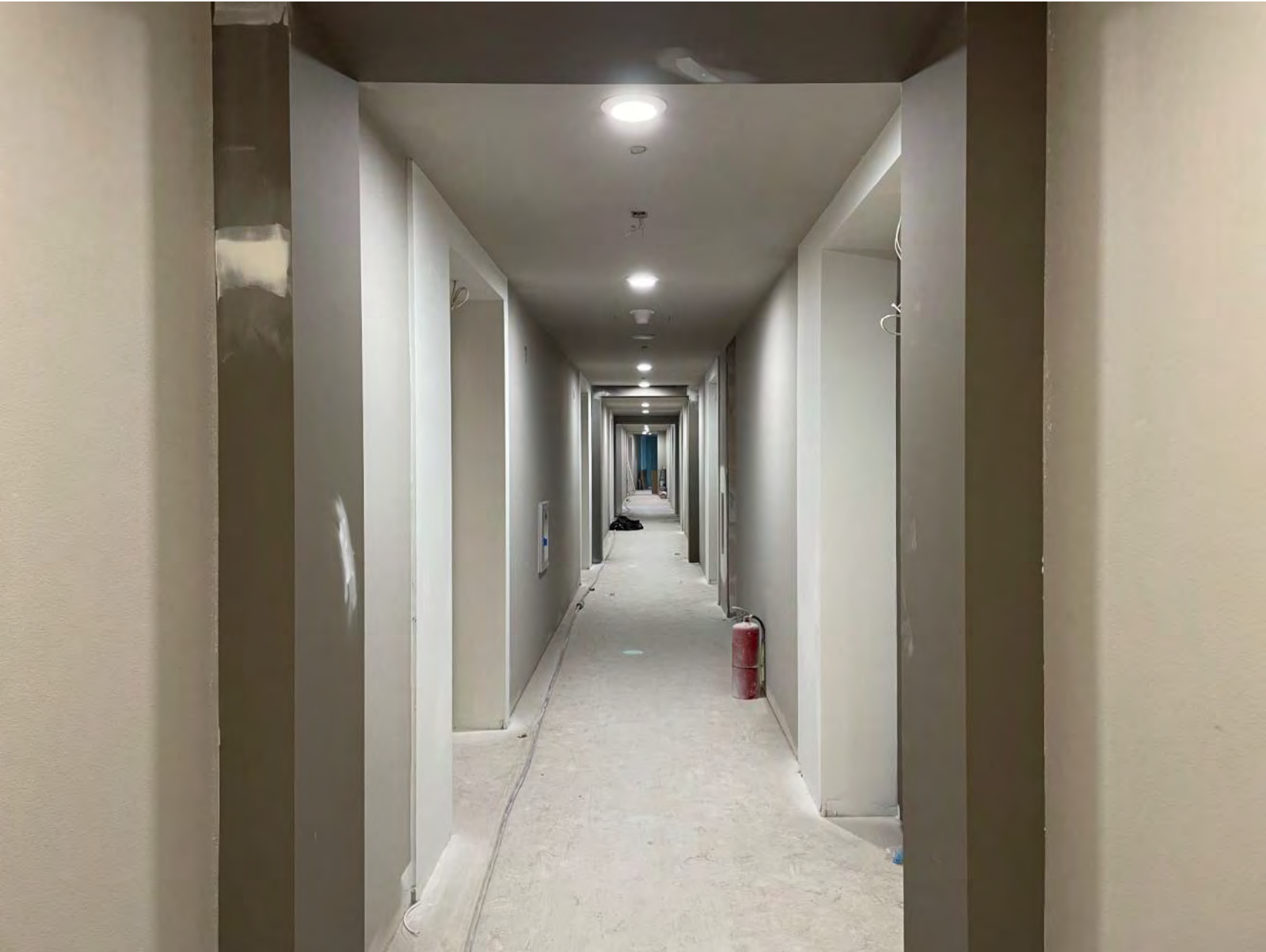
Phase 1, Level 6 Corridor Touch-ups Ongoing
