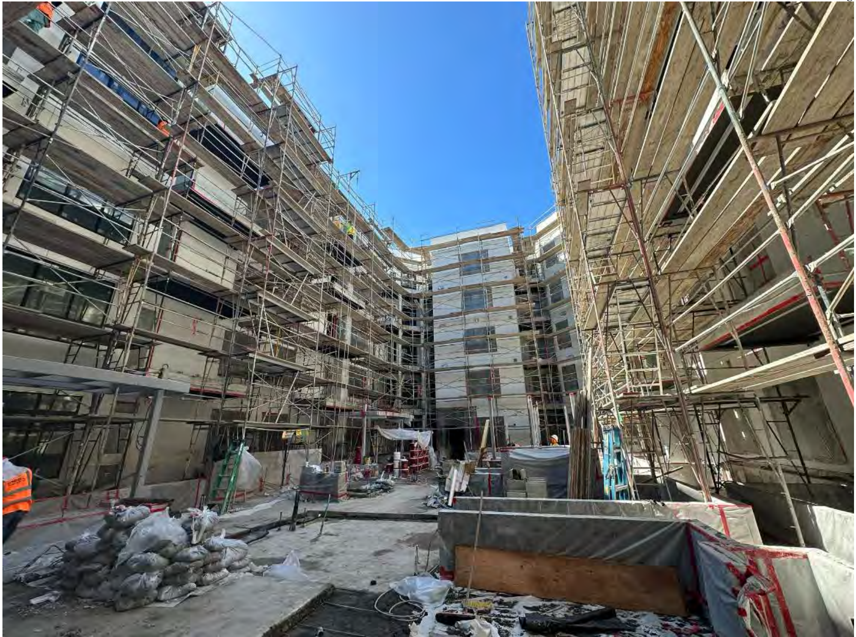
Ground View of Courtyard D
