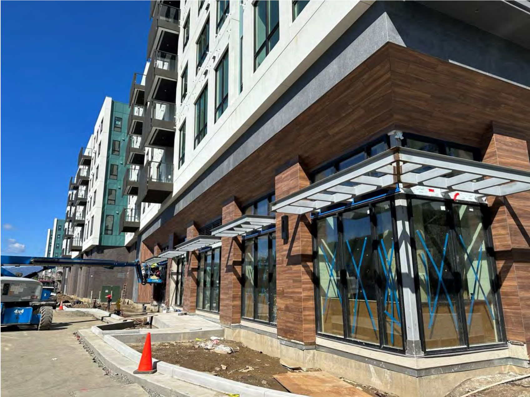
View of Southeast Storefront
