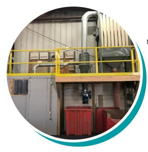
Modified disintegrator enclosure to help mitigate noise exposure when running and enhance roof structure walkability & OSHA compliance
