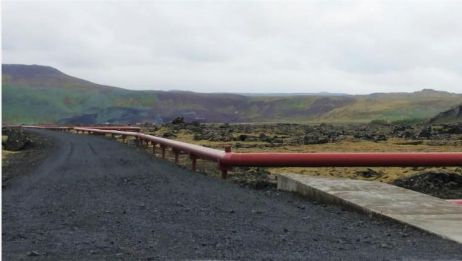
These large pipes transport very hot water from the geothermal areas to the cities. All the heating of buildings is done by this geothermal energy
