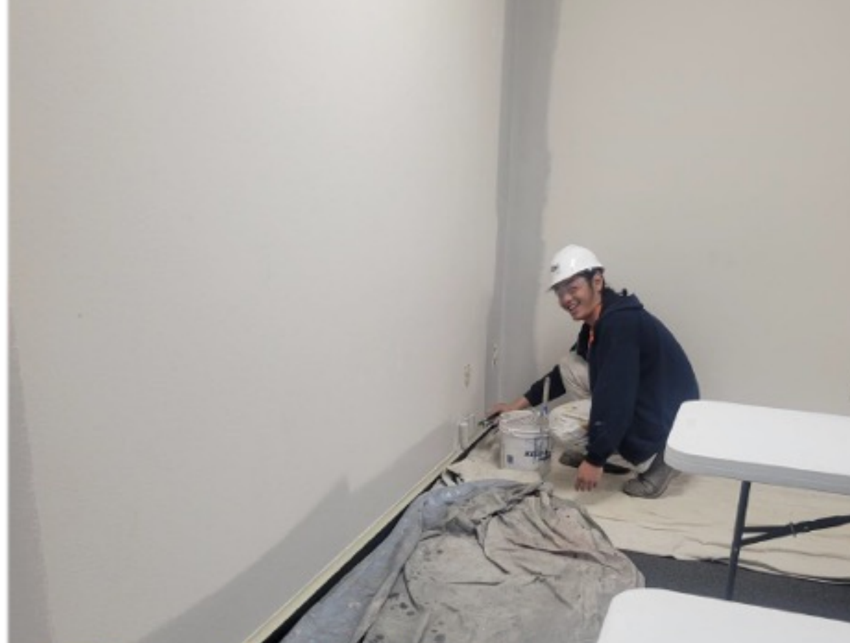
ABC NorCal Painting Apprentice Billy Her cutting in the walls at the ABC NorCal Sacramento Training Facility.
