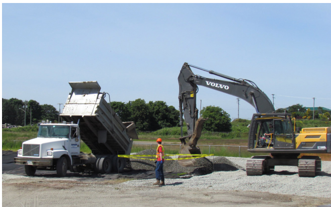
Crews placing aggregate in a laydown area for the McLoughlin Point Wastewater Treatment Plant in Esquimalt.
