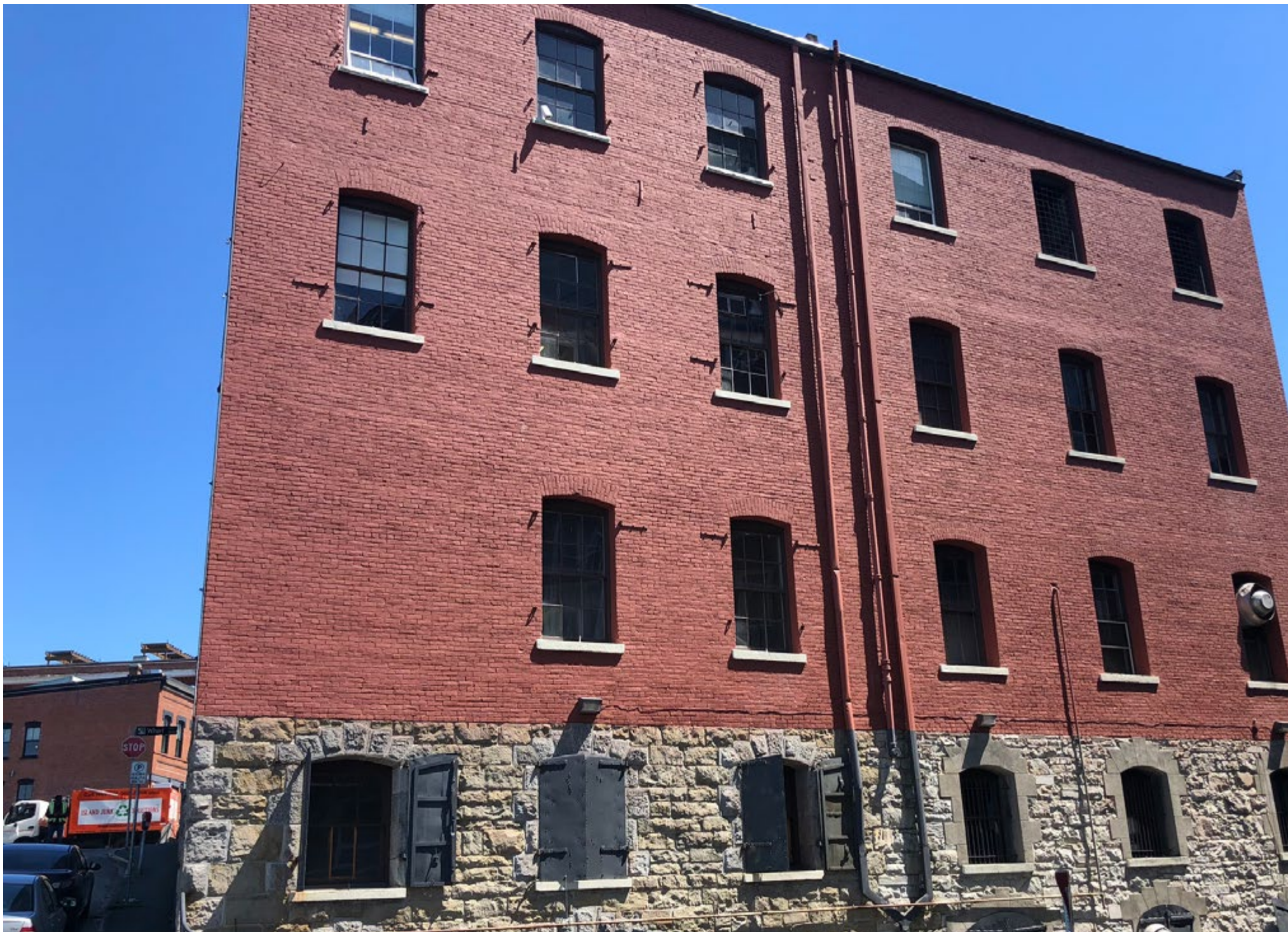
VIEW OF HARBOUR FACING FRONTAGE
