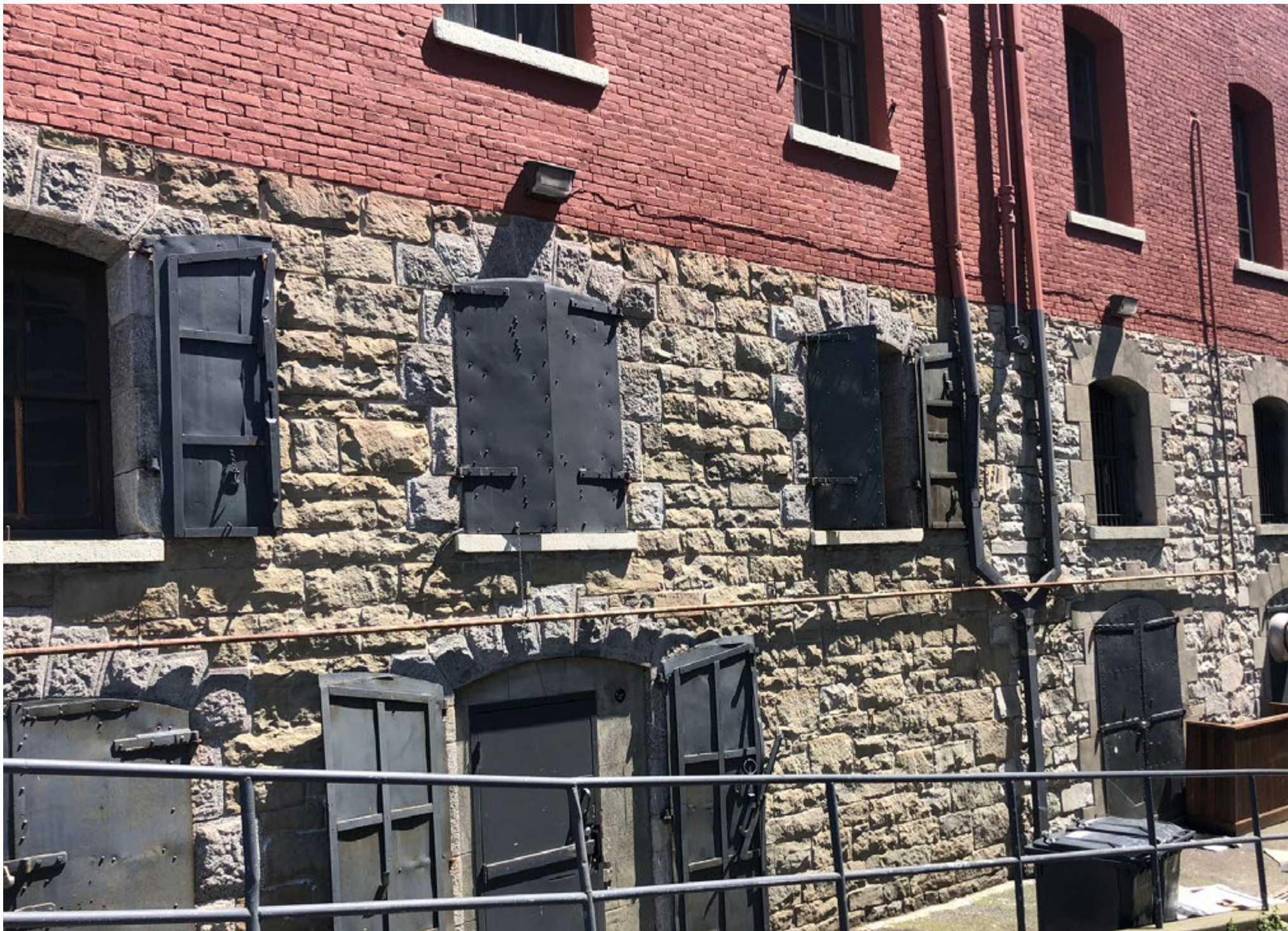
DETAIL VIEW OF LEVEL 1&2 HARBOUR FACING FRONTAGE
