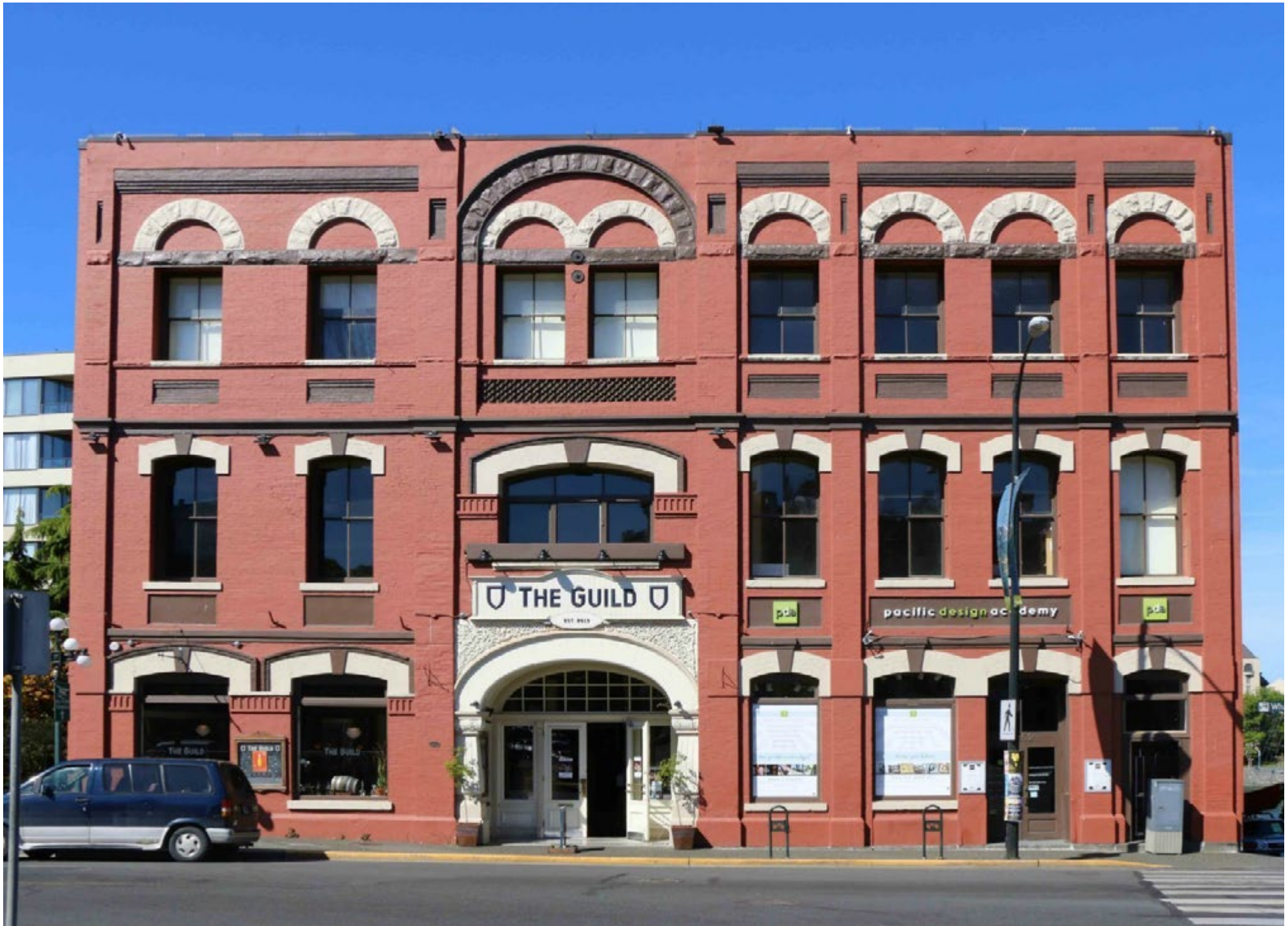
VIEW OF WHARF STREET FRONTAGE
