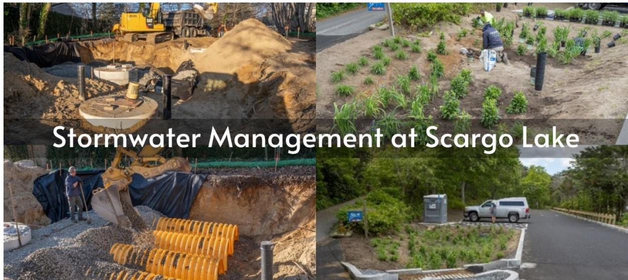
Above: Installation of underground infiltration chambers and water quality unit at 6A Landing (left) and native plantings at Dr. Lord's Road Scargo Beach bioretention area (right) (Credit: Gerald Beetham).
