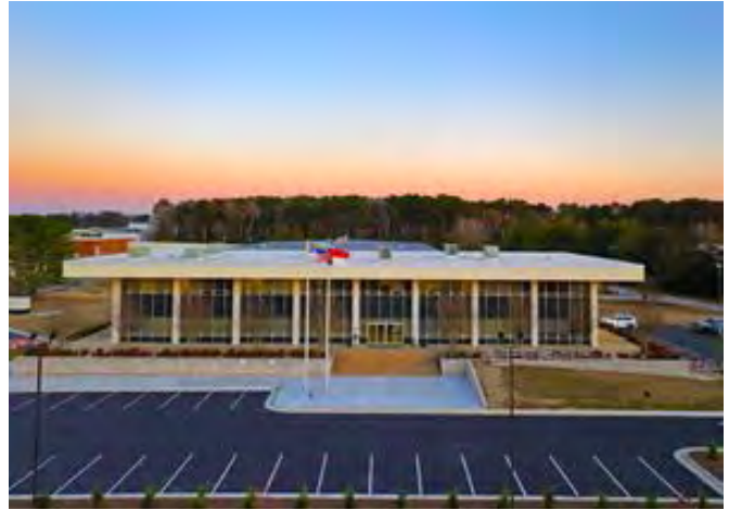
Recently Remodeled County Building
