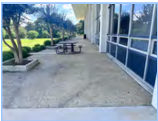
Admin Building Existing Exterior Sidewalk
