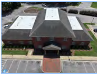
Tax Office Roof
