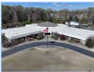
AG Center HVAC
