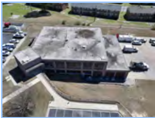
Emergency Services Existing Roof
