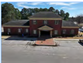
Tax Office Parking Lot
