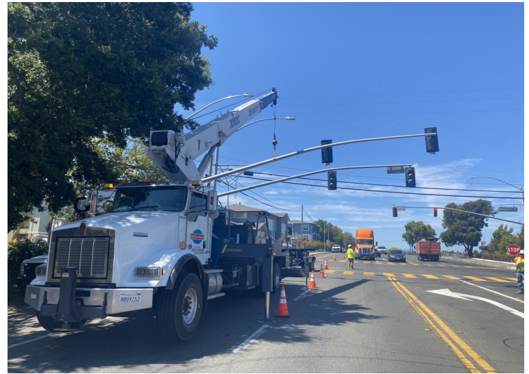
(New light signal being installed)
