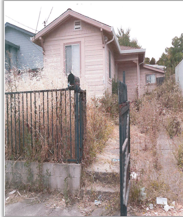
Overgrown Dry Weeds
