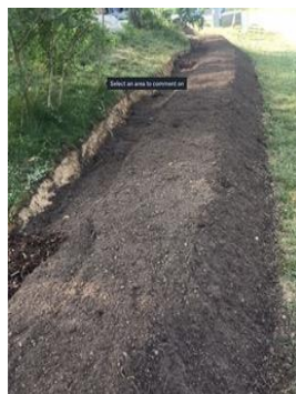
The swale is empty and the topsoil is on the berm
