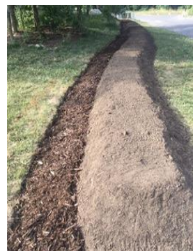
Swale filled with wood chips; berm covered with topsoil.
