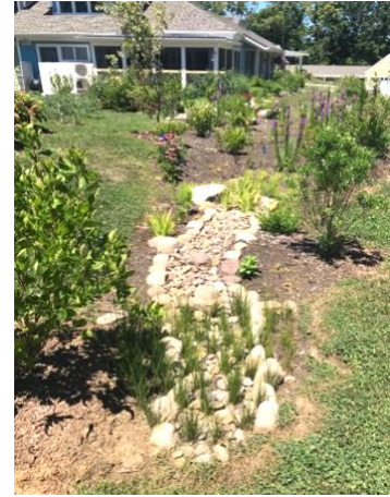
The largest of three rain gardens that help to catch and absorb rains, slowing down runoff while nurturing native plants.
