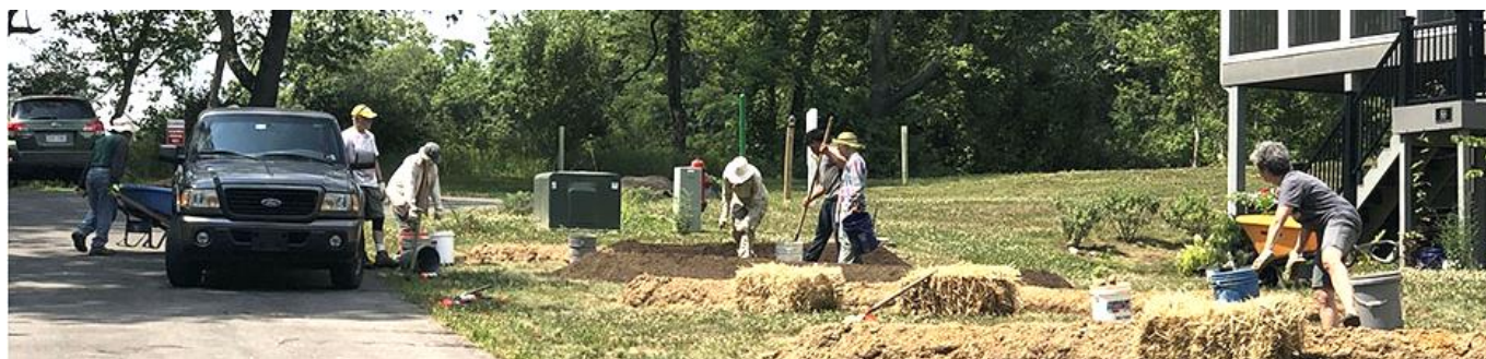
It takes a village. Here you can see the berms that are below the swales. The berms will be covered with topsoil and the swales are being filled with wood chips. The wood chips will absorb the water and retain it. They will be a water source for the trees when they are planted.
