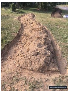
The swale is first dug by the machine
