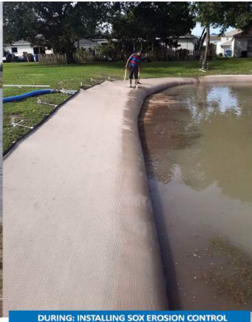
DURING: INSTALLING SOX EROSION CONTROL
