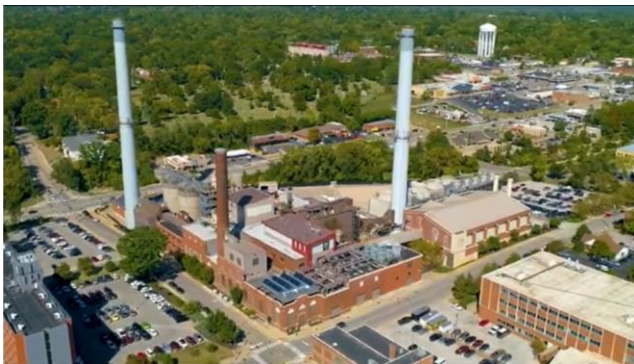
Figure 1: University of Missouri Power Plant (Source: University of Missouri)
