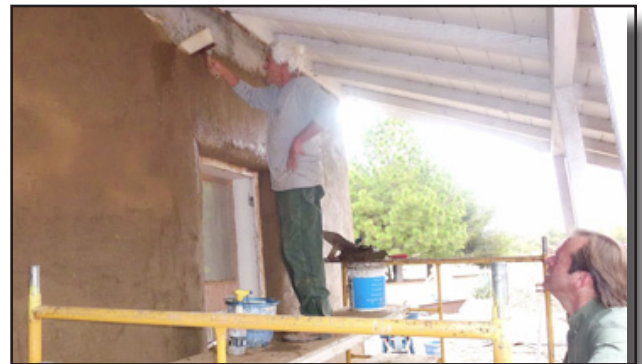
Exterior restoration of Las Flores Carriage House
