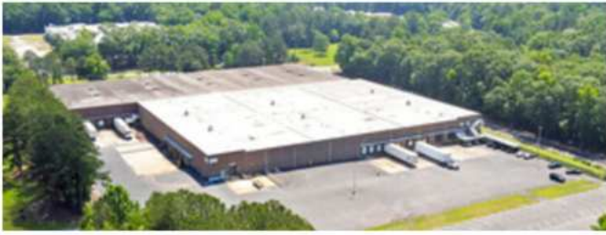
LEASED | 188,610 SF WAREHOUSE AT 4801 CARGO DRIVE COLUMBUS, GA 31907
