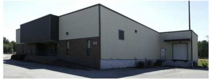
LEASED | 5,000 SF WAREHOUSE AT 153 CHALLENGER COURT COLUMBUS, GA 31904
