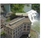
**#7 View of hydro plant** - This building houses three turbines, which together generate 46 MegaWatts of electricity, enough to power over 30,000 homes. Known as Station 5, this hydro plant began operating in 1917. To reach the turbines, water flows down a 2,000-foot-long tunnel. The tunnel begins upstream, at a rack house above the Middle Falls, which you'll see later in this tour.
