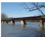
**#6 Erie Lackawanna Railroad Bridge** - This bridge was constructed in 1915 to carry the Rochester branch of the Erie Railroad over the Genesee River. The heavy plate girder structure is supported by cut stone piers. It was converted into a pedestrian bridge in 2011 and now links the University of Rochester's River Campus and Rochester's 19th Ward.
