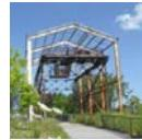
**#5 Coal chute** - This metal structure was part of a facility which unloaded coal from railroad cars. At the bottom of the chute, conveyors moved the coal to a manufactured gas plant and to Beebe Station, a coal-fired power generating facility.
