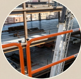
Steel Frame Erection
