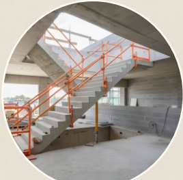
Concrete Pours and Finishes
