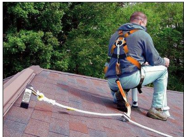
Miller Claw Permanent Roof Anchor, RA45
