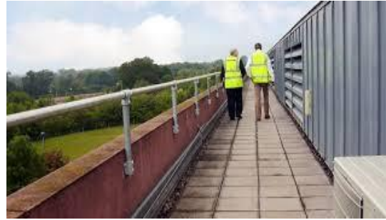
Mounting a railing directly to the top of a roof parapet is a cost-effective way of providing rooftop perimeter fall protection
