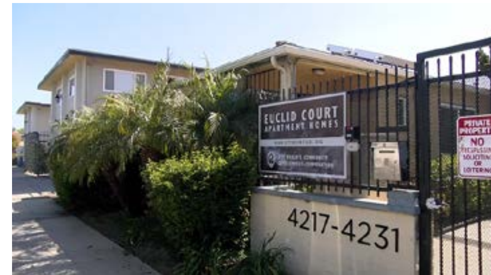
Euclid Court Apartments, an affordable housing complex in City Heights is pictured on May 27, 2021.
