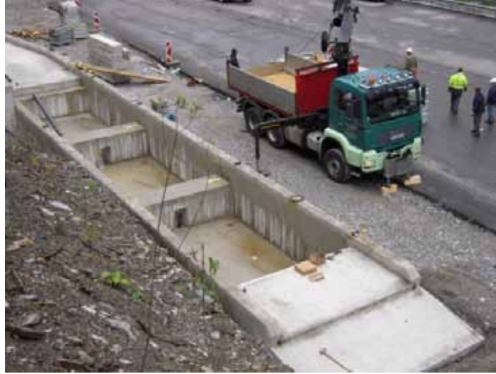
The scale foundation should include adequate approaches that comply with local regulations
