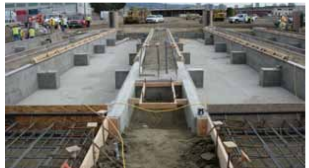
Foundation preparation can take place prior to the scale components arriving on site
