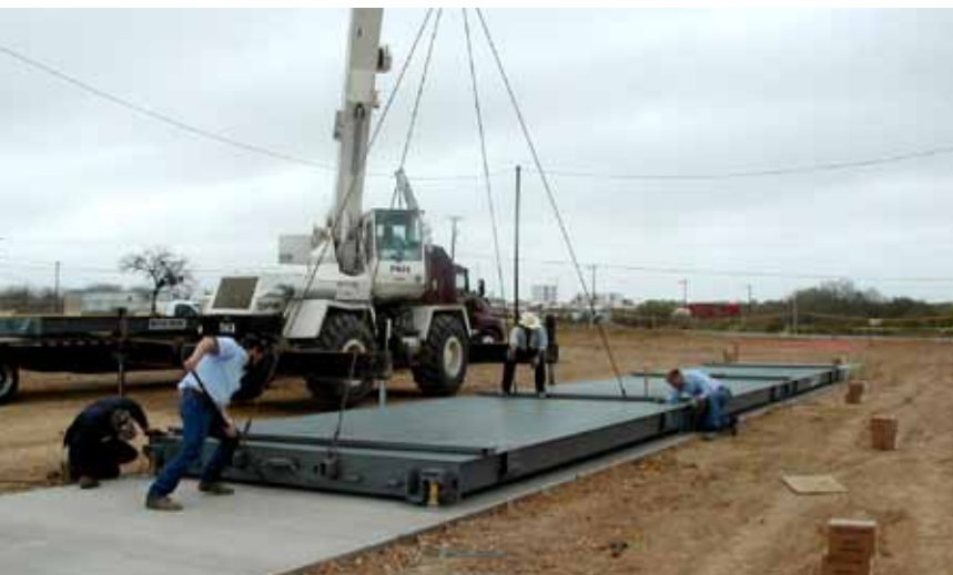
A steel deck weighbridge is installed
