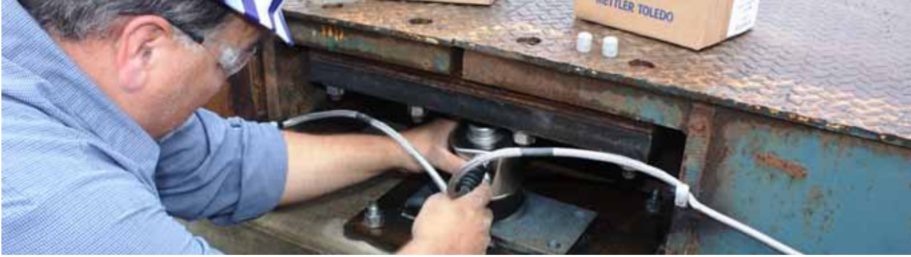
Upgrading an existing weighbridge by installing a new load cell system enhances the scale's accuracy and reliability
