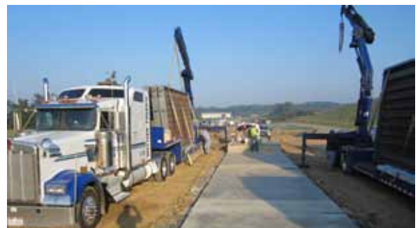
Specially designed delivery trucks are able to transport the weighbridge modules upright
