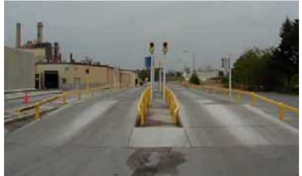
Scale-mounted guiderrails are attached to the side of the weighbridge modules with bolts or welded brackets
