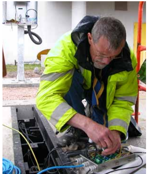
A technician tests load cell cable connections inside a junction box
