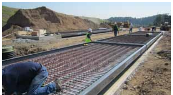
This scale is nearly ready for concrete to be poured into the deck modules
