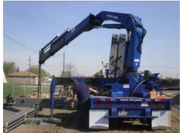
Piecing together a portable frame truck scale on a prepared compacted soil site
