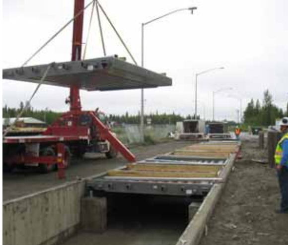
A pit-style scale is placed in an excavated foundation, flush with the ground
