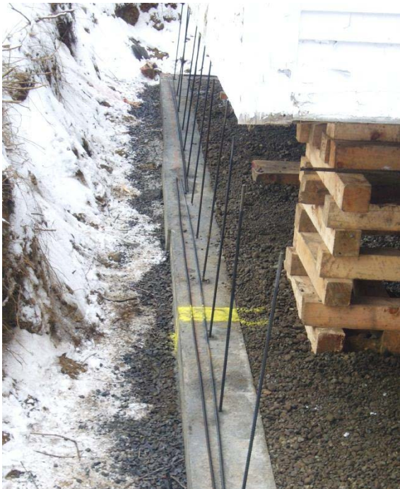
Construction photographs - December 2016 - Former 1881 Union Church in Adirondack - for Museum Use Church was 'suspended' on cribbing & I-beams and now is sitting on its New Concrete Foundation!
