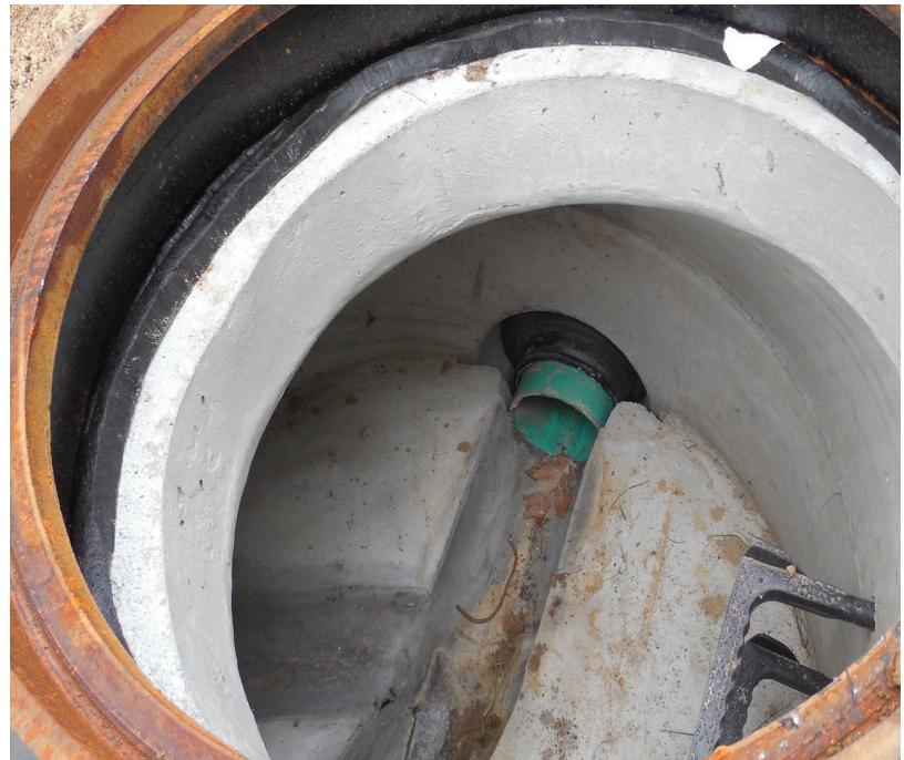
The same manhole as seen in 2022. No visible damage. The ConBlock MIC works.
