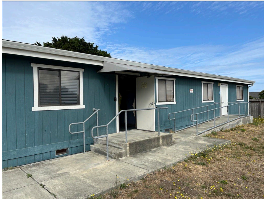
Photograph of Employee Entrance (left) and Public Entrance (right) to 752 South Franklin Street Office.
