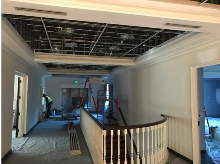
2nd Floor Lobby
