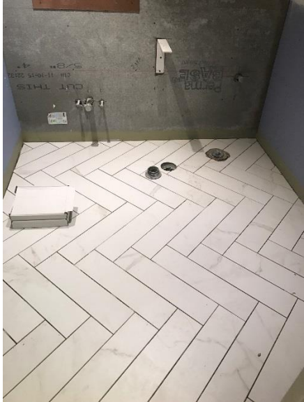
1st Floor Women's Restroom
