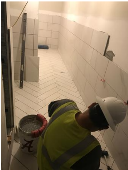
2nd Floor Women's Restroom
