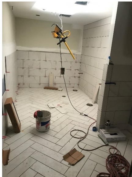
2nd Men's Restroom
