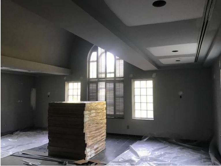
2 nd Floor Tilson Room
