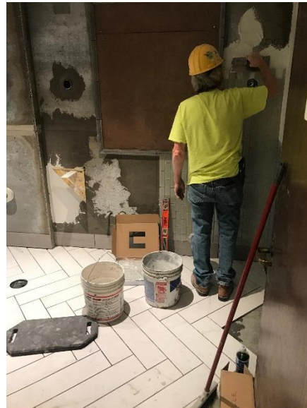
1 st Floor Family Restroom
