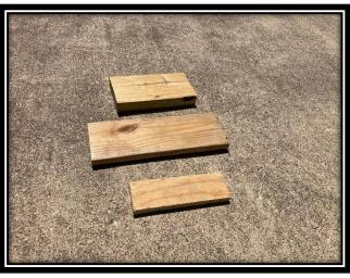
The reason I carry these scraps is to better determine the right threshold ramp solution, particularly in cases where a door will have to clear the completed transition ramp. I have had the experience of using a measuring tape to check door clearance, and then on build day finding an unexpected clearance issue. These boards give me a way to quickly evaluate options with readily available lumber thicknesses, either individually or in combination.
