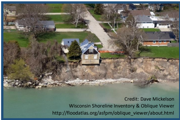
A house in Southeastern Wisconsin teeters over the edge of a bluff after coastal storms and waves eroded the shoreline 40 feet in four years.
