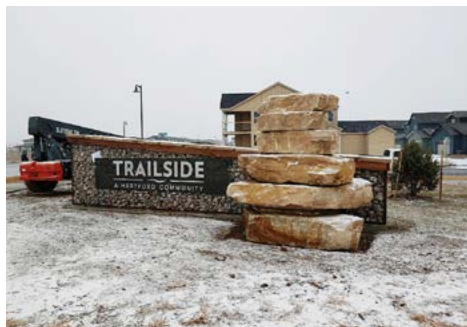
A gabion wall monument sign for Trailside, A Hartford Community in Colorado.
