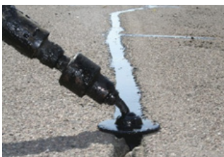
Routed crack being sealed
