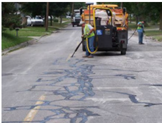
Crack sealing in the field
