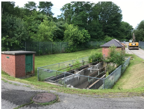
Figure 1: Bearbrook CSO before removal.
