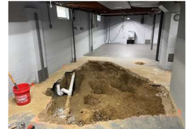
Figure 6. Remediation of the Foundation
