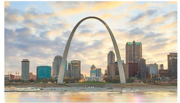
The arch's two legs were built separately, and if their measurements were off by as little as 1/64th of an inch, they would not have been able to join at the top.
