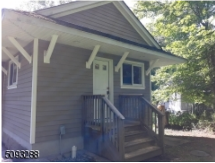
PORCHES RECENTLY STAINED
