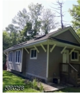
5 SKYLIGHTS, 2 OPEN REMOTELY
