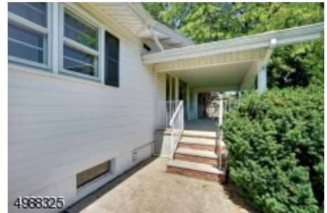
VINYL SIDING, WRAPPED SOFFITS!
